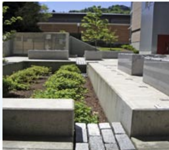
University of Portland — roofwater runs into splash boxes, through block runnels and planter beds, then into underground storage for re-use.
