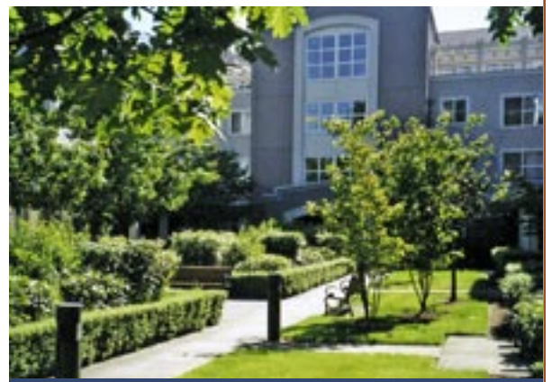
Buckman Heights Apartments — courtyard raingardens infiltrate runoff from downspouts and walkways.
