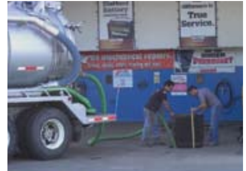
Collection of trucked liquid waste
