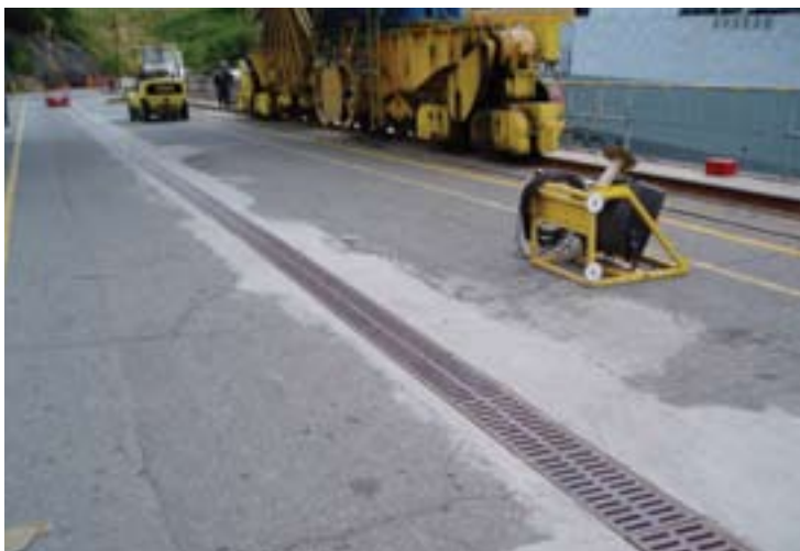
Grated trench drains
