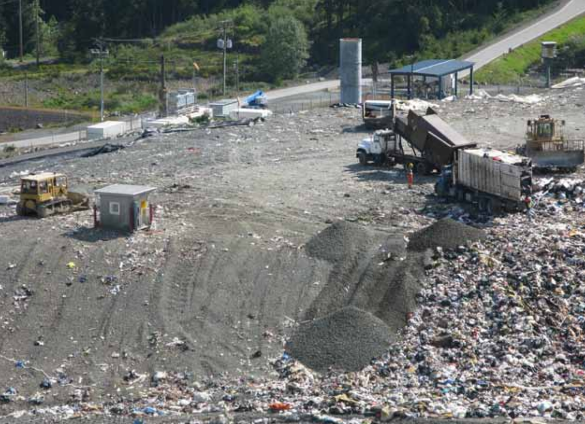
The active face area and gas utilization area at Hartland landfill.
