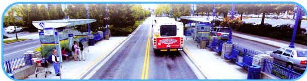
Median Busway on No.3 Road in Richmond
