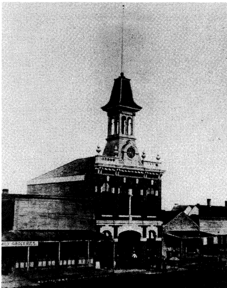
Deluge Fire Hall, Victoria, Yates Street
