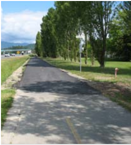
New pavement on Lochside Trail
