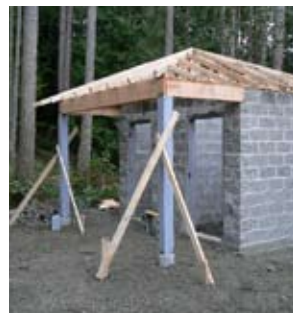
Aylard Farm toilet building - East Sooke Regional Park
