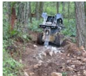
Phelps connector trail construction - Thetis Lake Regional Park
