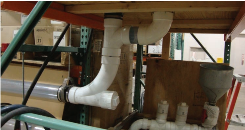
PHOTO 4-E PLUMBING UNDER FLUSH STAND
