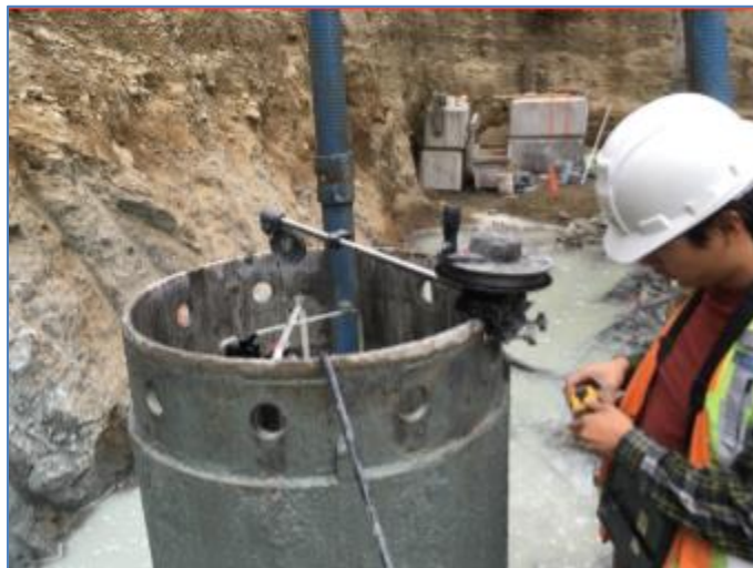
Figure 29– Arbutus Attenuation Tank –Video Inspection of Secant Pile.
