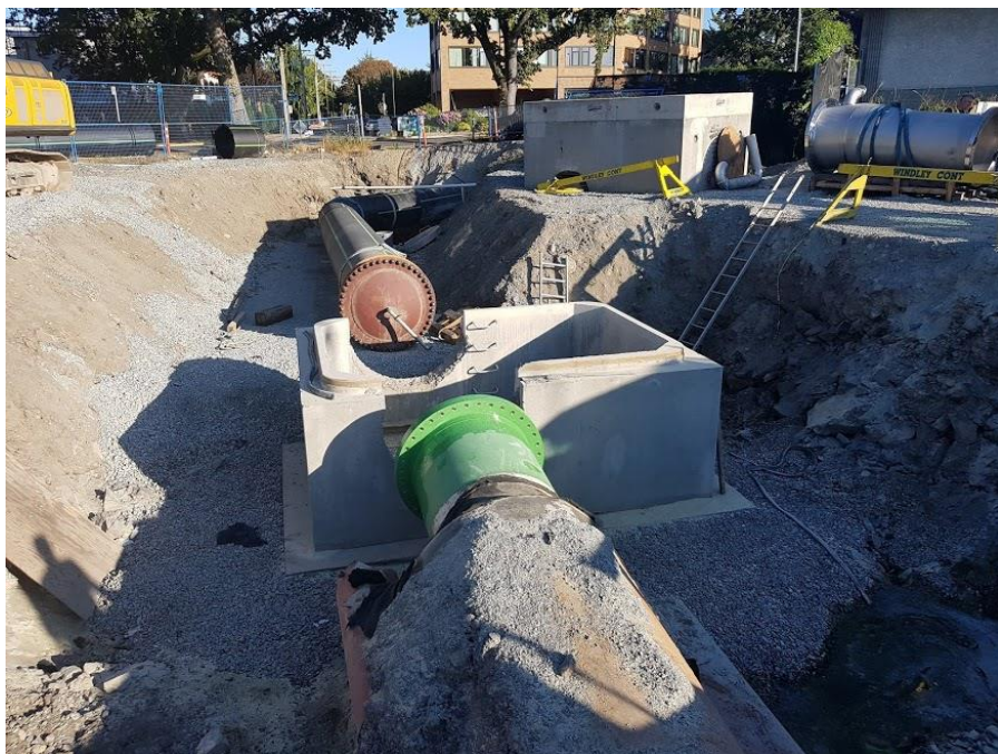
Figure 18–Clover Forcemain- Flange coating complete on under harbour pipe.
