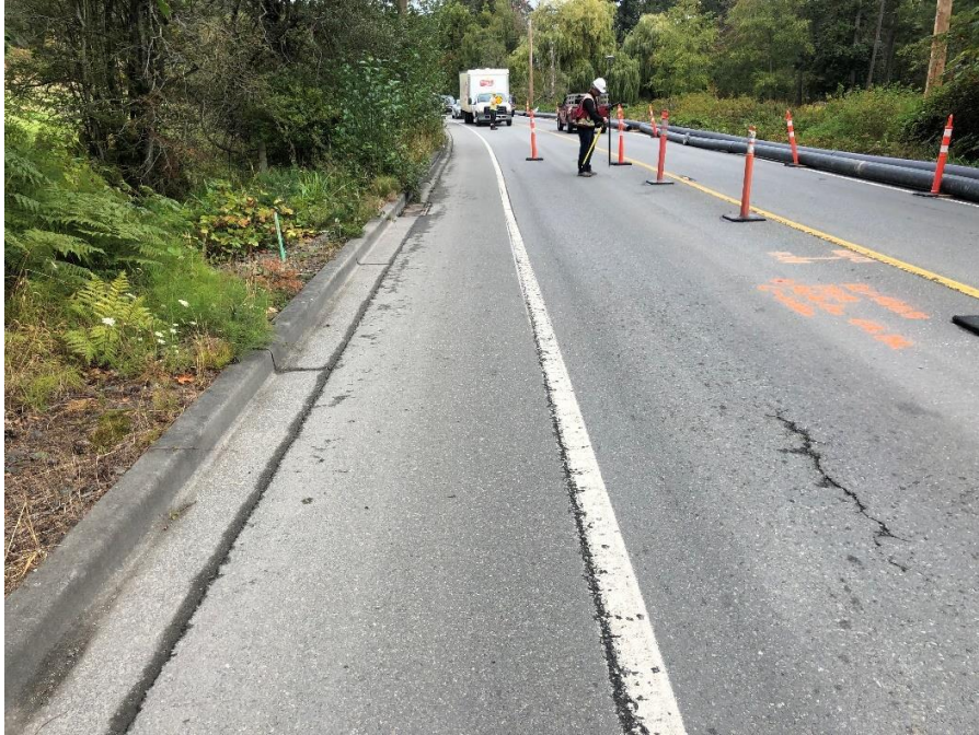
Figure 23–Residual Solids Conveyance Line- Layout of pipe alignment on Interurban Road.
