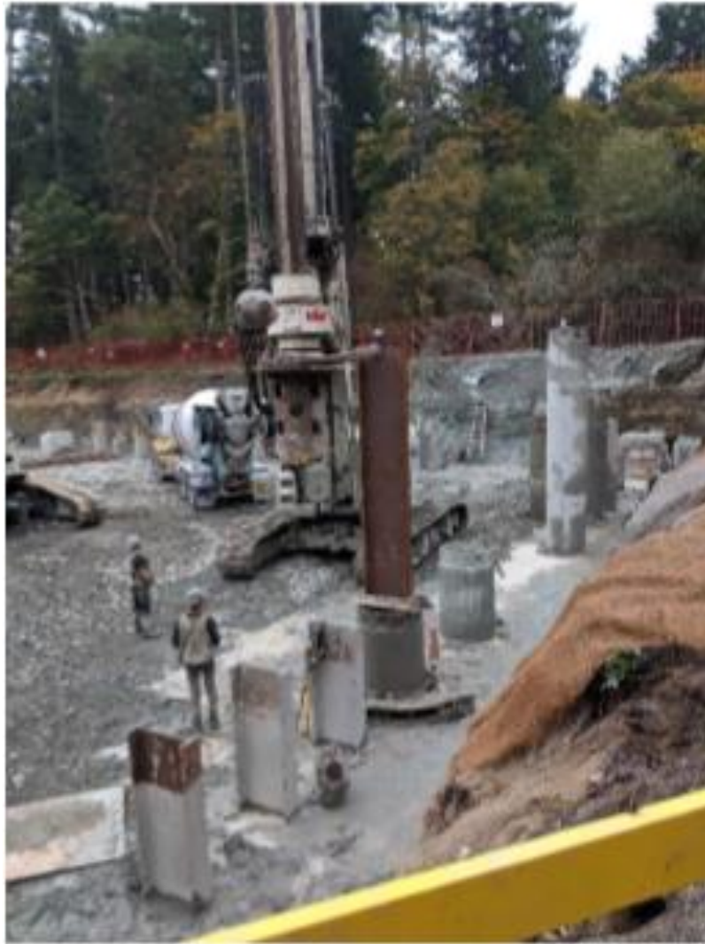
Figure 28–Arbutus Attenuation Tank- Installation of Reinforcement for Secant Pile.
