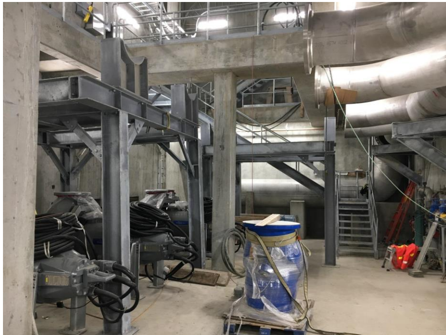
Figure 12–Clover Point Pump Station- Installing pump room pipe supports.
