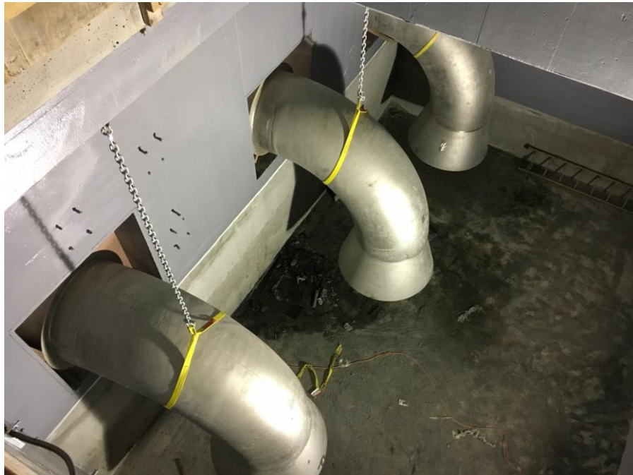
Figure 11–Clover Point Pump Station- Setting storm suction spoils.
