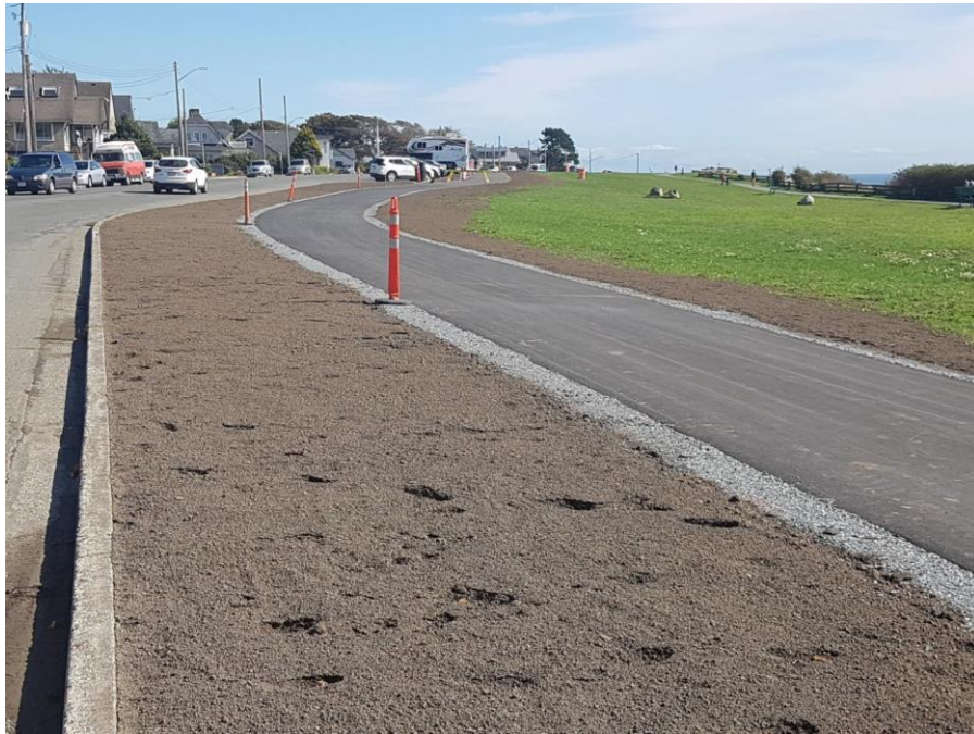
Figure 19–Clover Forcemain–Cycle track paved and landscaping in progress.
