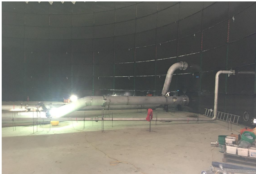
Figure 10– Residuals Treatment Facility- Installation of interior piping inside Digester 2 ongoing.
