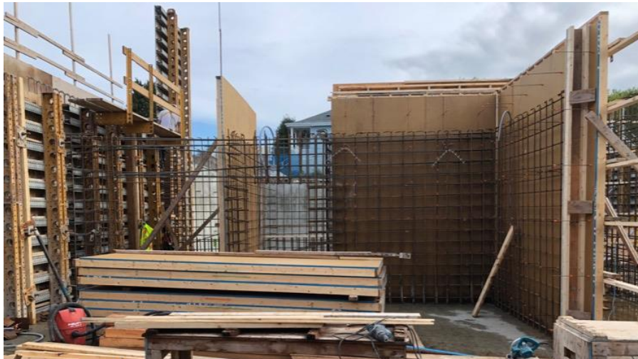
Figure 16-Macaulay Point Pump Station- Installing formwork for genset room wall.
