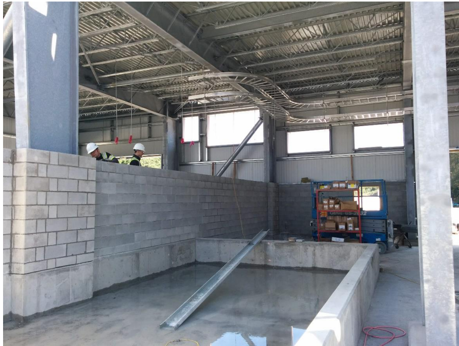
Figure 7- Residuals Treatment Facility- Installing concrete block walls in Residuals Handling Building.
