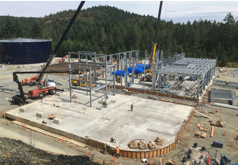
Progress at the Residuals Treatment Facility
