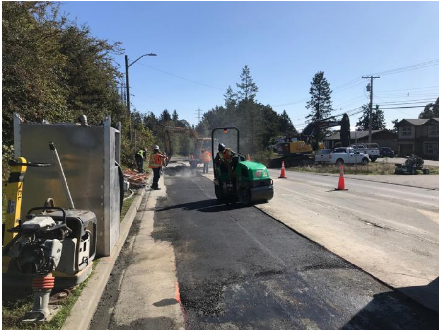
Figure 24–Residual Solids Conveyance Line- Lower course paving on Interurban Road.
