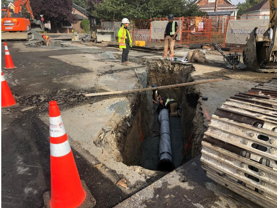
Figure 21–Residual Solids Conveyance Line- Trench excavation and pipe installation at Gore Street.
