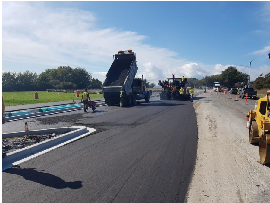
Figure 17–Clover Forcemain-Ogden Point - Road restoration in progress.
