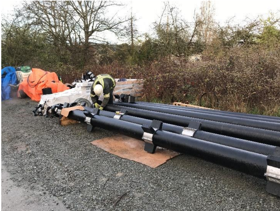
Figure 22–Residual Solids Pipes – Installing spacers on highway crossing pipe.
