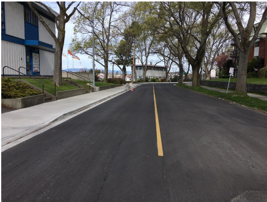
Figure 19–Clover Forcemain- Top lift of paving Niagara Street to Dock Street.
