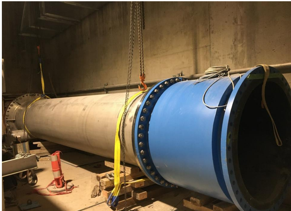
Figure 15-Macaulay Point Pump Station- Stainless steel pipe installation to Forcemain.
