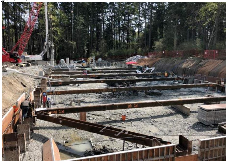
Figure 26–Arbutus Attenuation Tank–Installed diagonal and lateral struts atop the secant piles.
