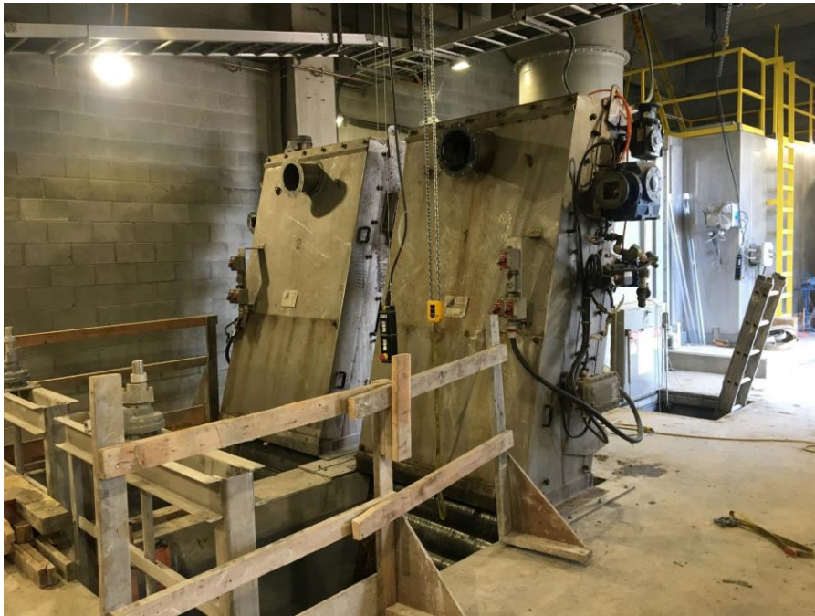
Figure 11–Clover Point Pump Station- Existing screen installation to new inlet channel.
