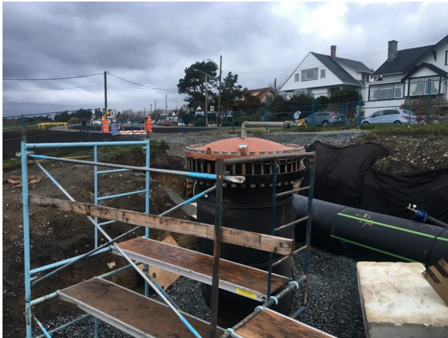
Figure 13- Clover Pump Station – Forcemain pressure test.
