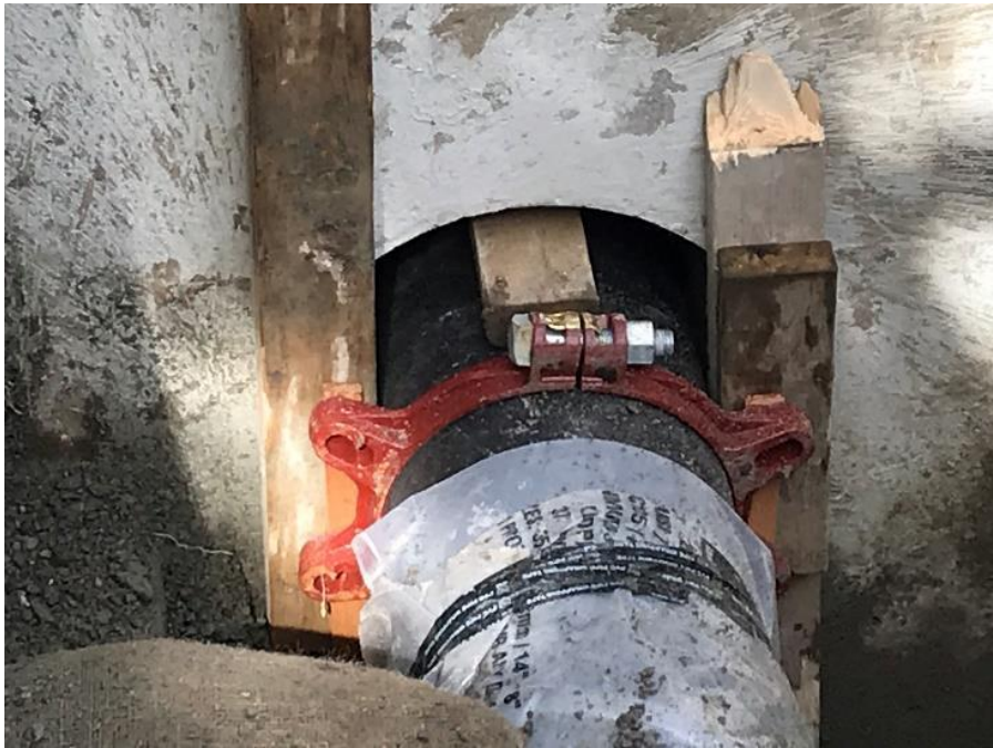
Figure 21–Residual Solids Pipes- Installation of pipe through Tillicum Bridge abutment.
