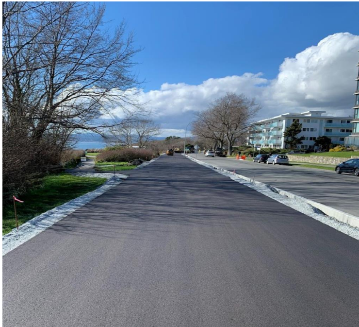
Figure 16–Clover Forcemain- Cycle track/road restoration from Government to Lewis Street.
