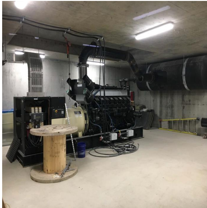
Figure 14-Macaulay Point Pump Station- Genset room progression.
