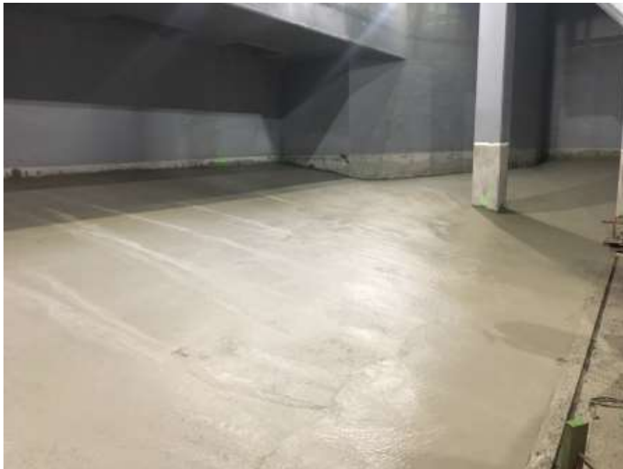
Figure 13–Clover Point Pump Station- Storm wet well benching.
