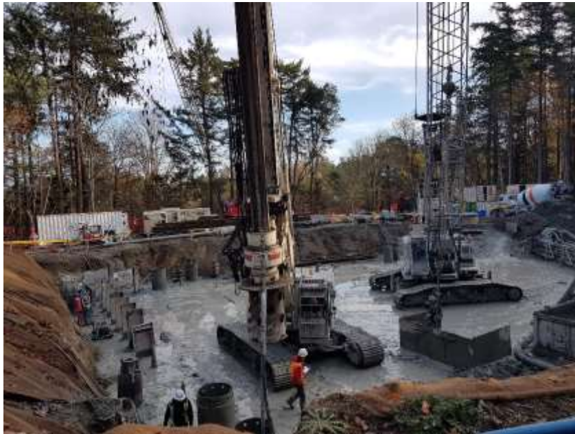
Figure 28–Arbutus Attenuation Tank- Installation of Secant Piles.
