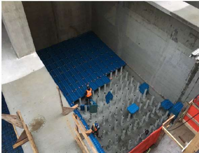
Figure 6– McLoughlin Point Wastewater Treatment Plant- Installing Monofloor soffit in BAF cell 3
