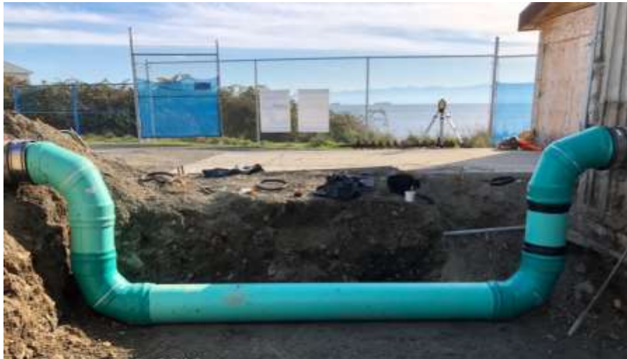
Figure 16–Macaulay Point Pump Station- Lowering vent pipe for construction of ramp.
