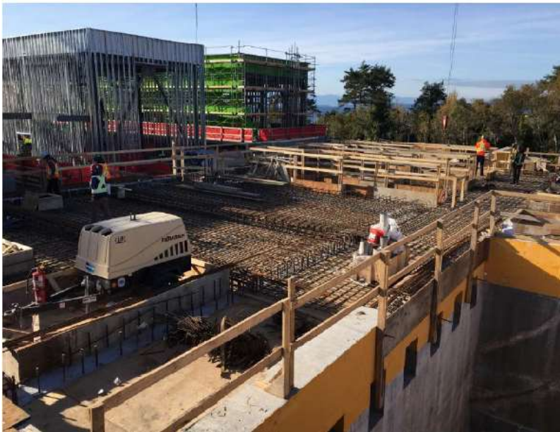
Figure 5- McLoughlin Point Wastewater Treatment Plant-Installing reinforcing steel in Dirty Backwash slab
