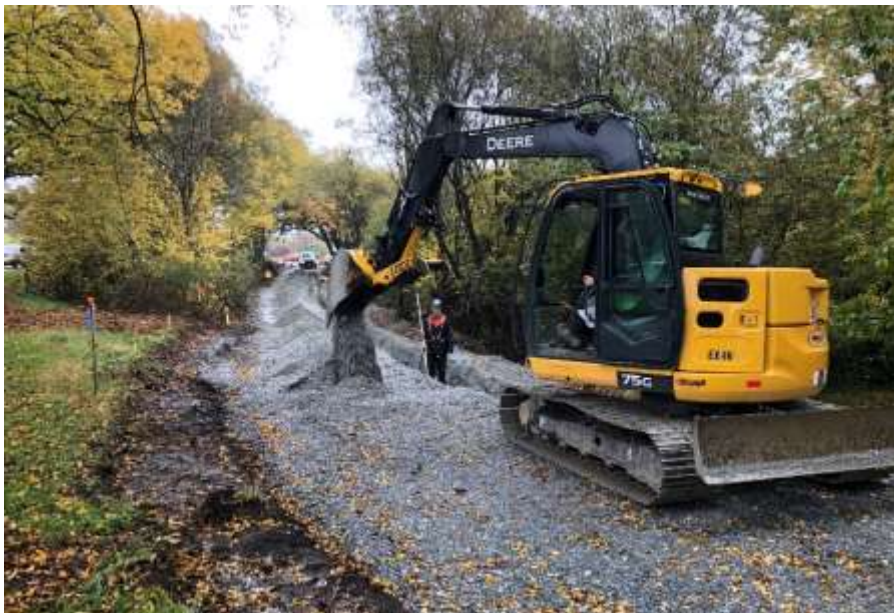
Figure 19–Clover Forcemain– Electrical conduit installs along cycle track corridor (foot of Douglas.)
