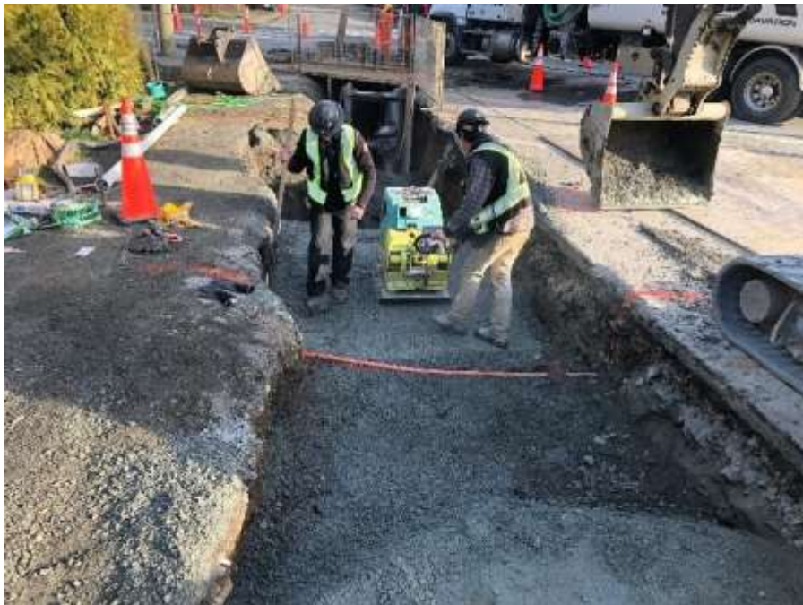
Figure 21–Residual Solids Conveyance Line- Backfill and compaction Grange Rd at Interurban Rd.
