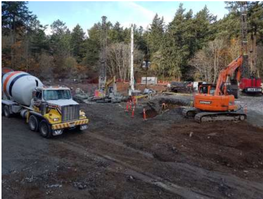
Figure 29– Arbutus Attenuation Tank –Site overview.
