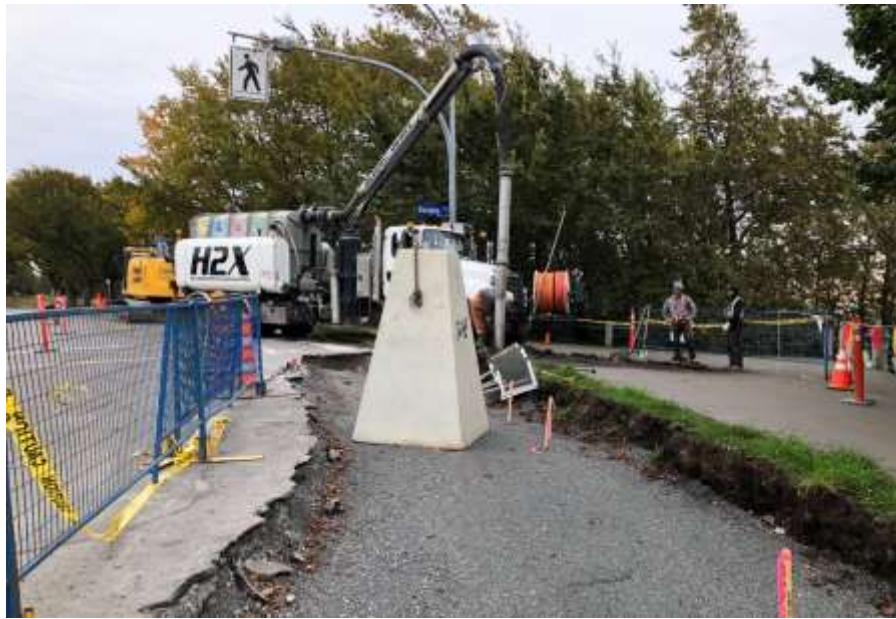
Figure 20–Clover Forcemain- New street light base installation at Dallas/Douglas Intersection.
