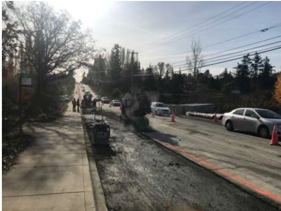
Figure 22-Residual Solids Conveyance Line- Asphalt over cut being completed on Interurban Rd.
