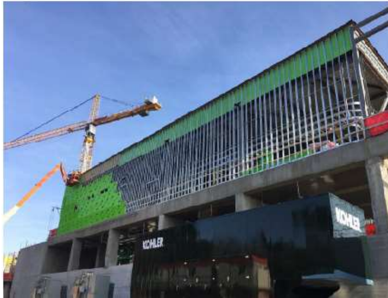
Figure 2– McLoughlin Point Wastewater Treatment Plant- Installing exterior sheathing on Electrical Room
