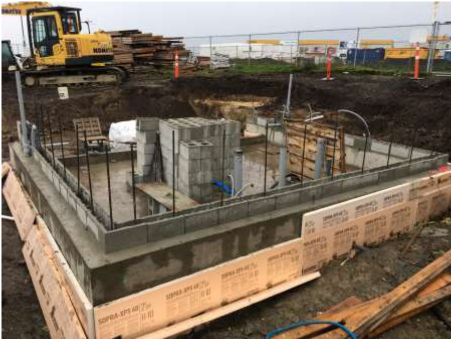
Figure 14- Clover Pump Station - Public washroom in progress.
