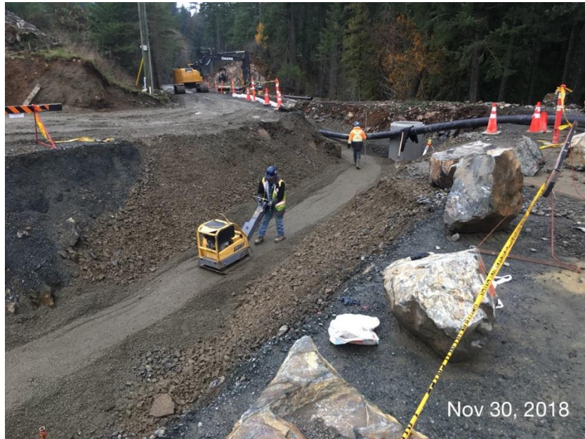
Figure 10 – Residuals Treatment Facility: preparation of bedding for Residual Solids Conveyance Line.
