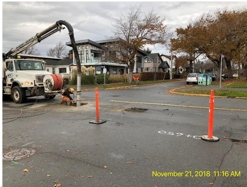
Figure 23 – Clover Forcemain: Dallas Road at San Jose Avenue, utility pre-locates.
