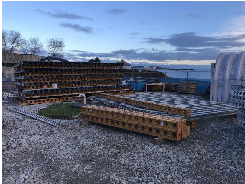
Figure 18 – Macaulay Point Pump Station: pre-fabrication of wall formwork.
