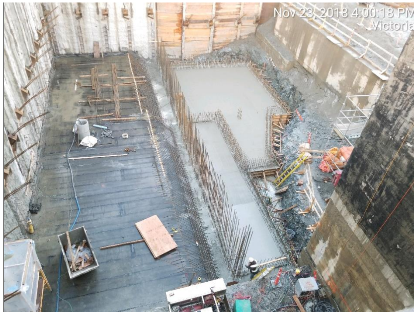
Figure 15 – Clover Point Pump Station: sanitary and storm wet well slabs complete.
