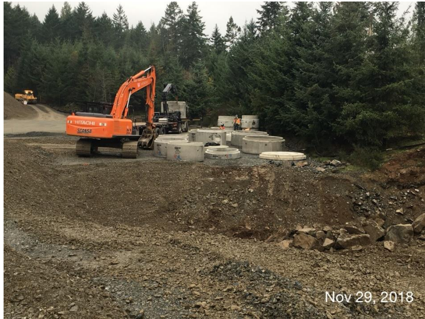
Figure 12 – Residuals Treatment Facility: components of Stormceptor STC3000 being delivered to site.
