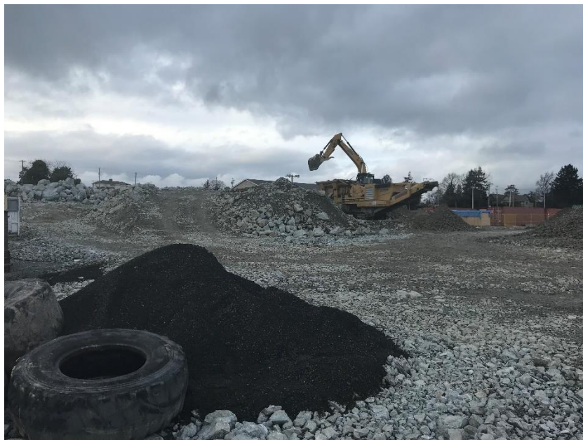
Figure 20 – Macaulay Point Pump Station: crushing of blast rock.
