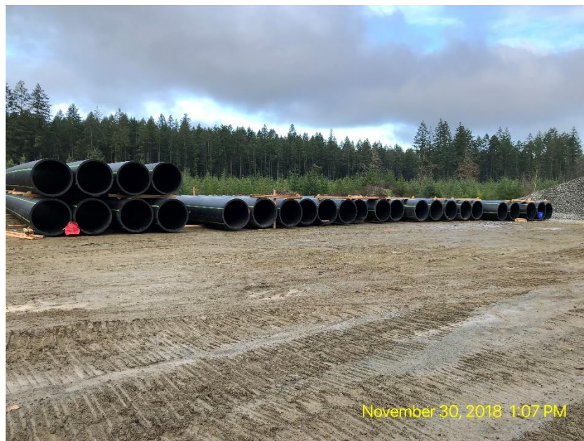
Figure 21 – Clover Forcemain: storage of HDPE forcemain pipe received.
