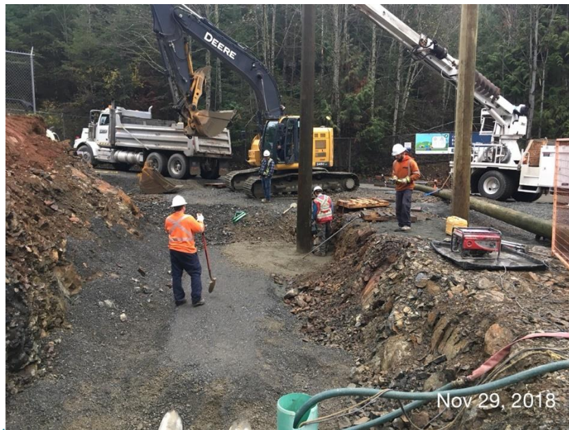
Figure 11 – Residuals Treatment Facility: erection of utility poles on main access road.
