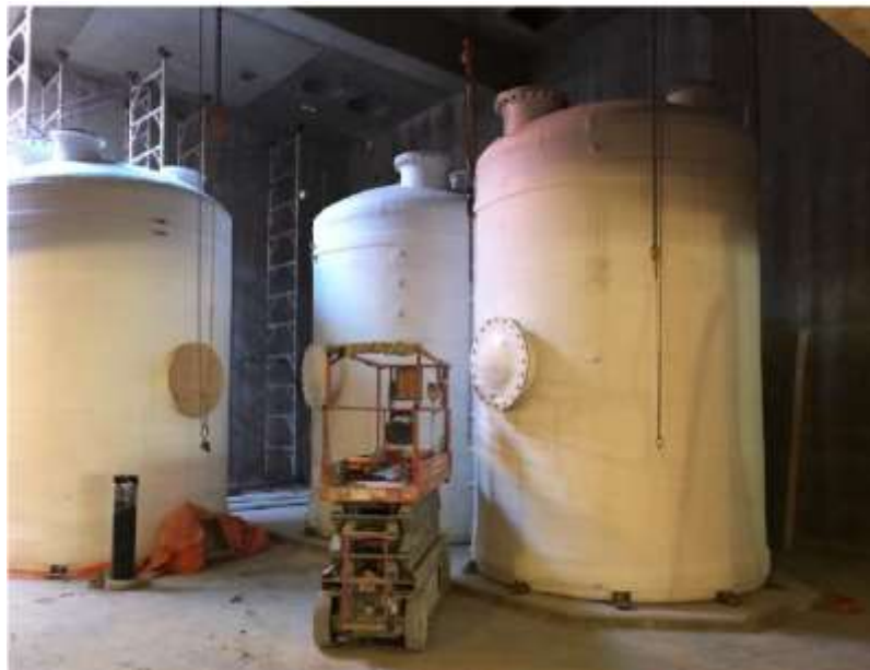
Figure 5– McLoughlin Point Wastewater Treatment Plant-Setting secondary odour control tanks.
