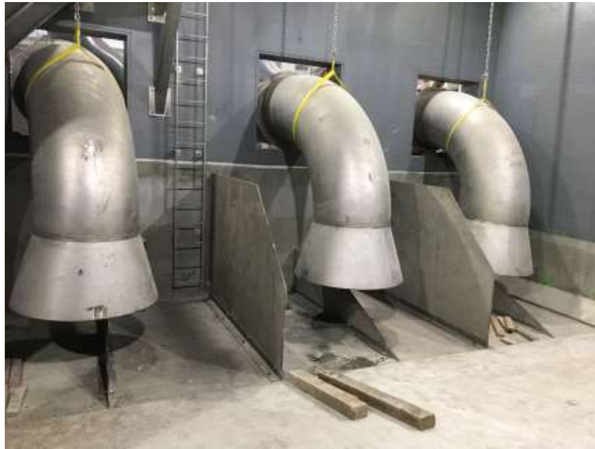
Figure 14- Clover Pump Station - Installation of suction spools.
