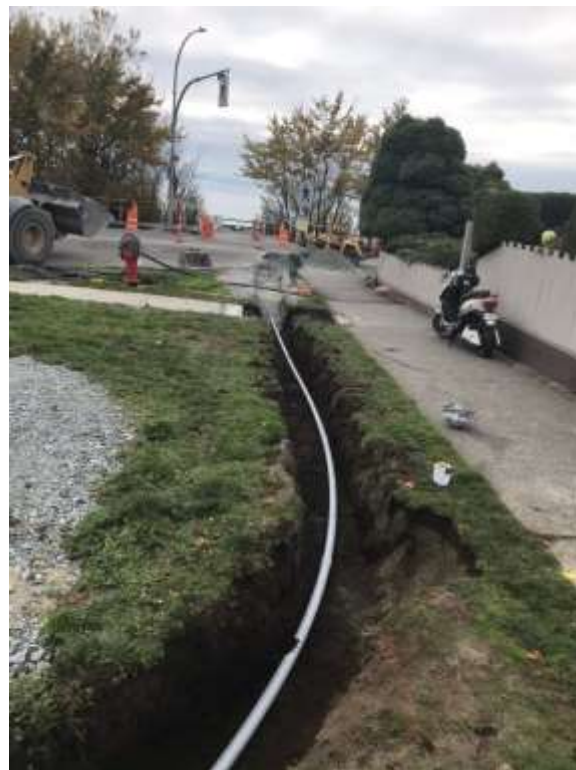
Figure 20–Clover Forcemain- Electrical conduit installation for lighting on Dallas Road.
