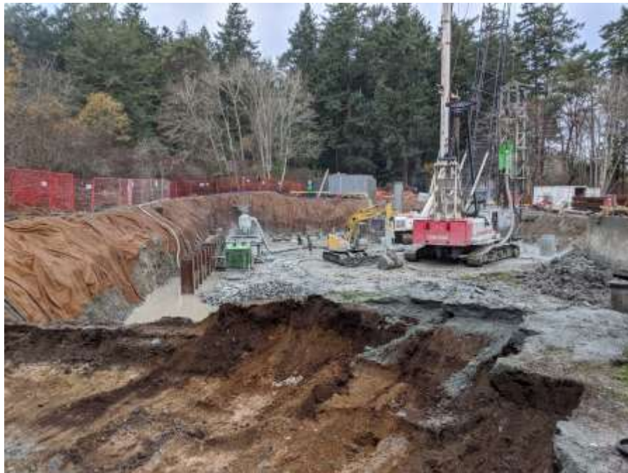
Figure 28–Arbutus Attenuation Tank- Ongoing secant pile wall drilling and installation.
