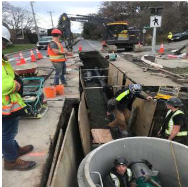
Figure 22–Residual Solids Conveyance Line- Line valve installation at Grange Road.
