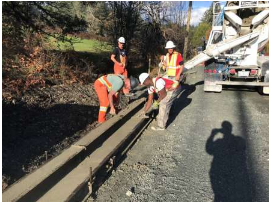
Figure 24–Residual Solids Conveyance Line- Curb replacement on Interurban Road near Goward Road.
