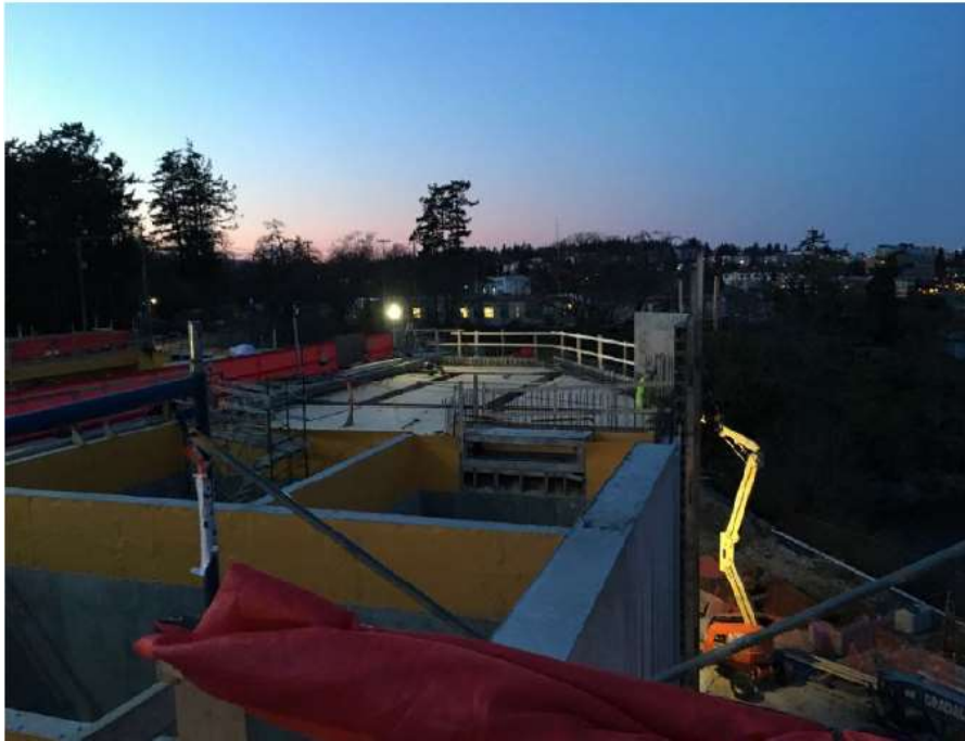
Figure 6- McLoughlin Point Wastewater Treatment Plant- Decking Odour control roof slab soffit.
