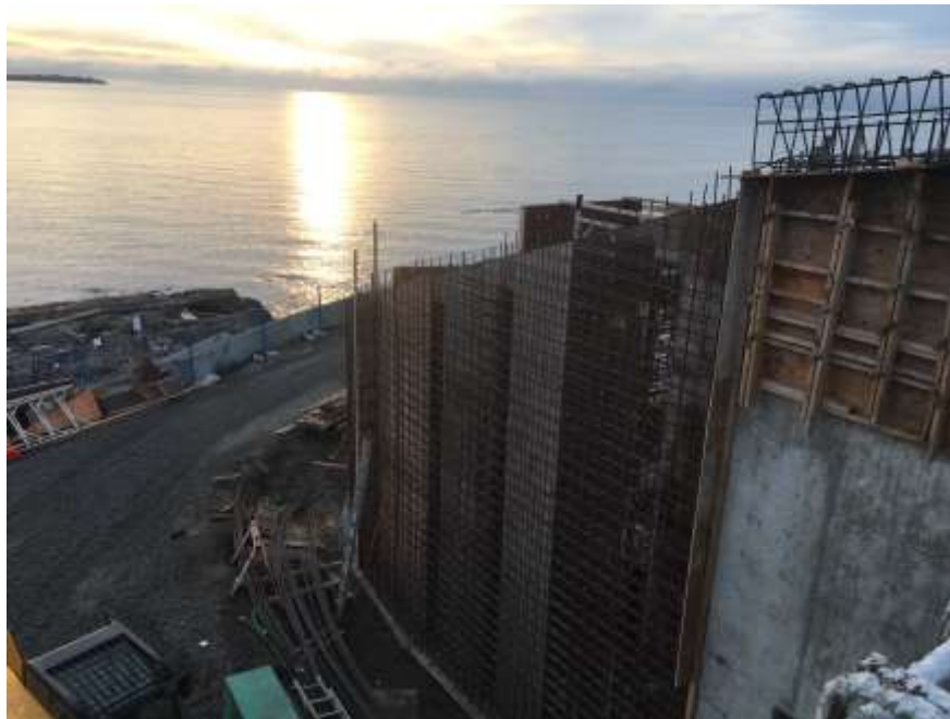
Figure 13–Clover Point Pump Station- Formwork and rebar for curved retaining wall.
