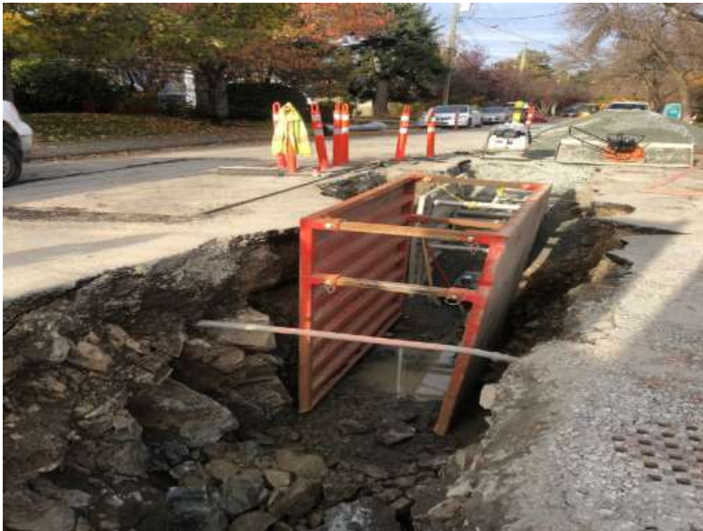
Figure 21–Residual Solids Conveyance Line- Pipe installation at Arm Street.
