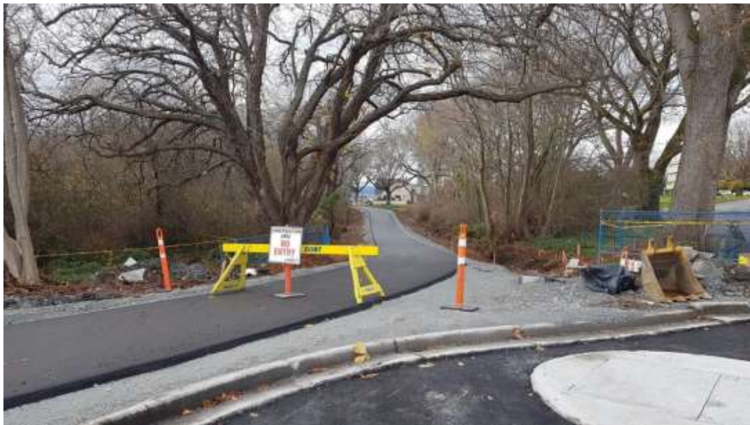
Figure 18–Clover Forcemain- Cycle track paving.
