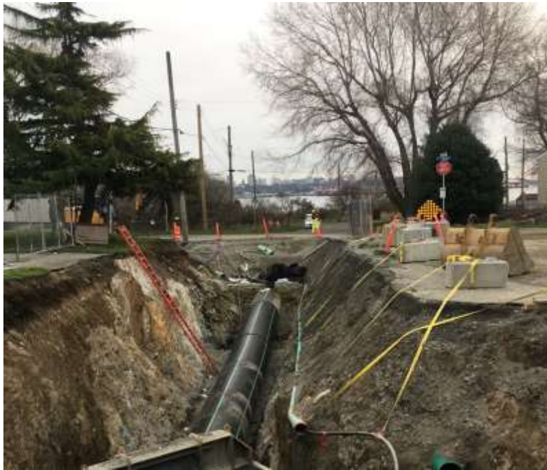
Figure 16—Macaulay Point Pump Station- 1350 mm forcemain installation along View Point Street.
