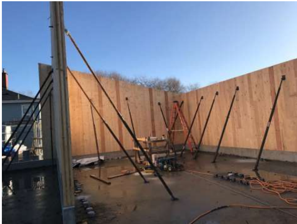
Figure 15–Macaulay Point Pump Station- Installation of cross laminated timber panels.
