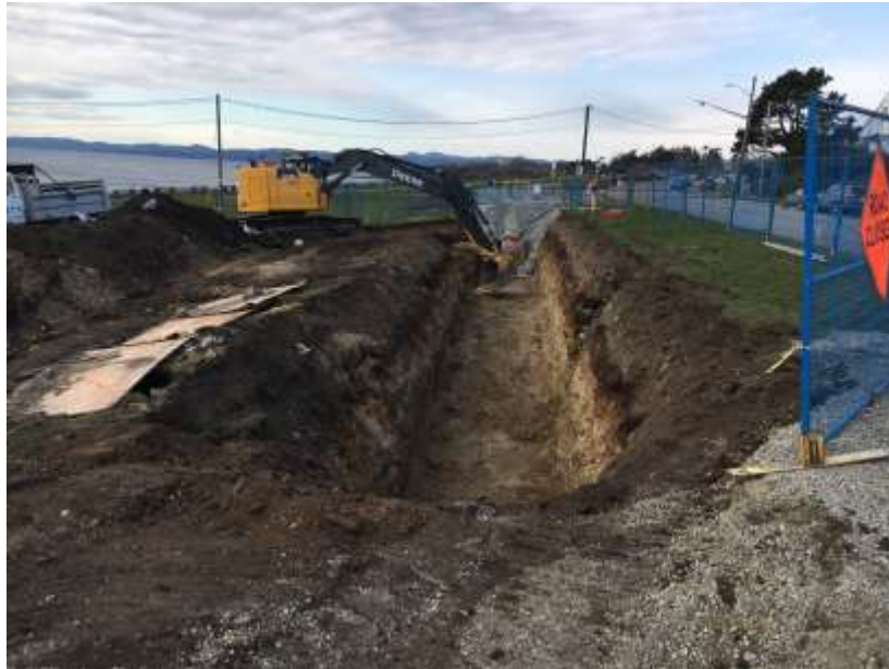
Figure 11–Clover Point Pump Station- Excavation for forcemain installation.
