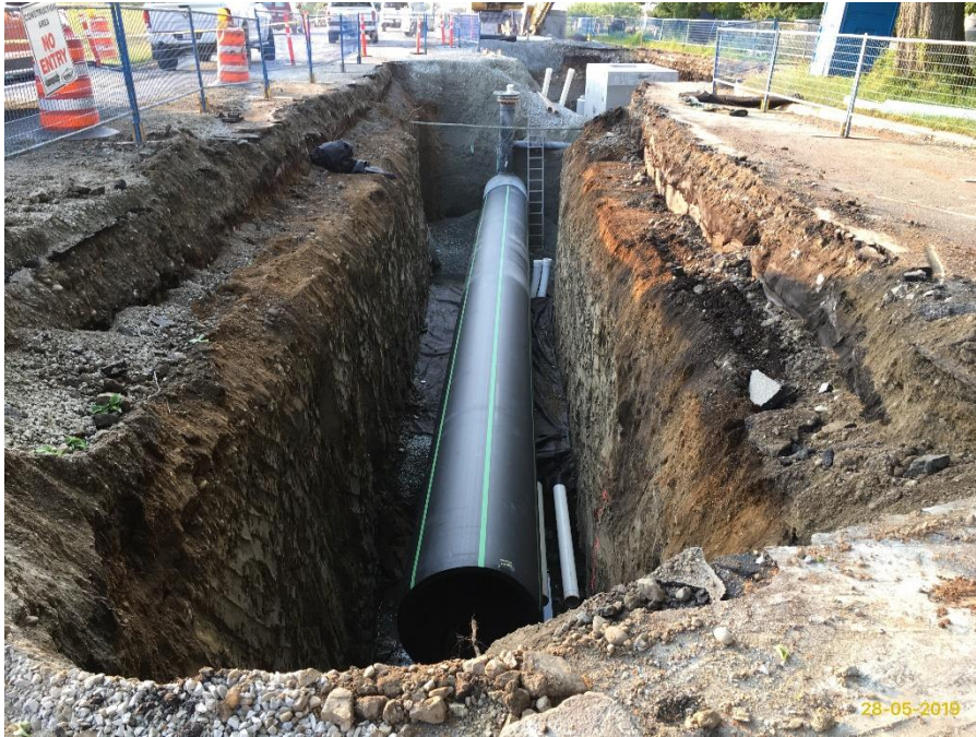
Figure 22 – Clover Forcemain: Installing forcemain towards Douglas Street.
