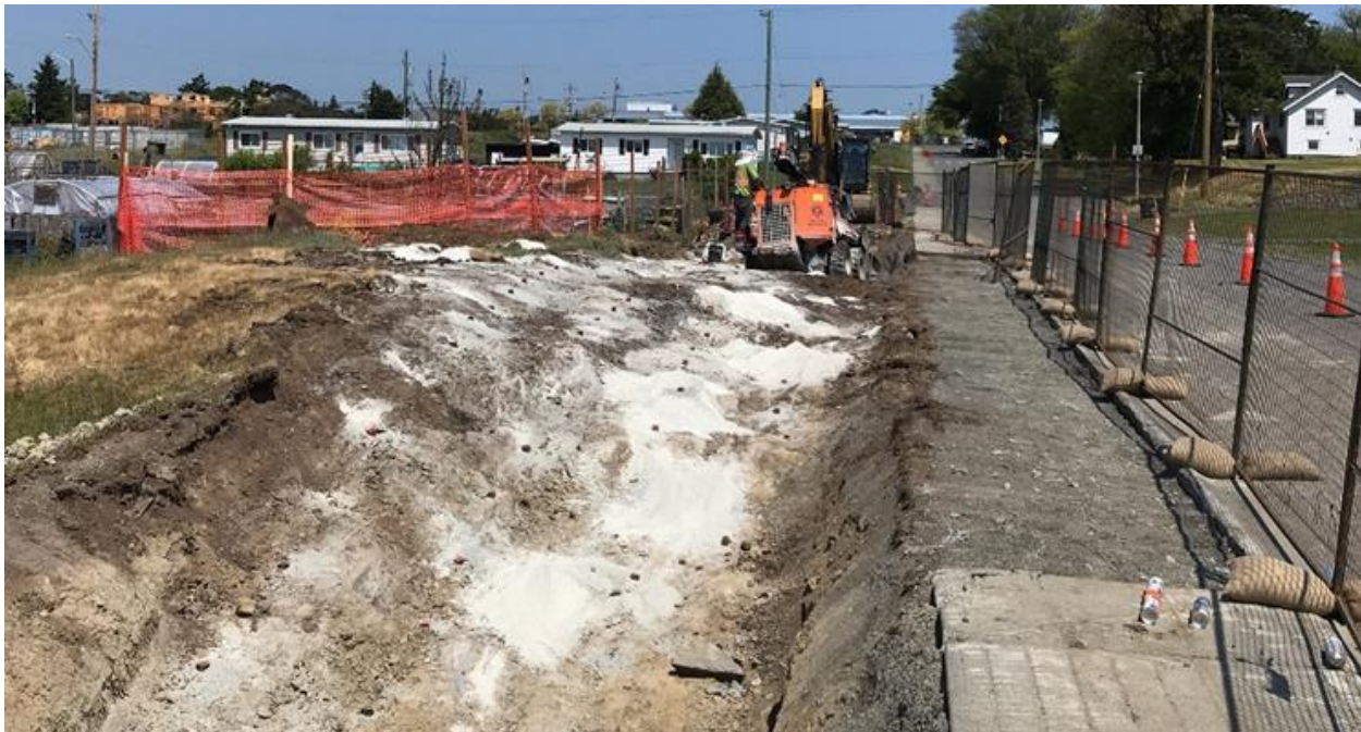
Figure 18 –Macaulay pump station & forcemain – drilling and blasting on Anson Street.
