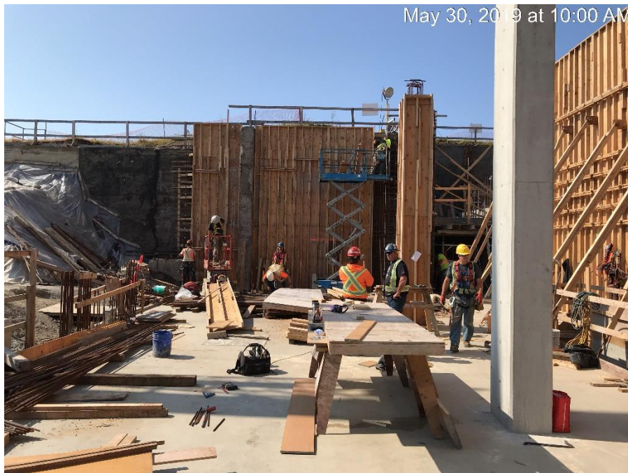
Figure 15 –Clover Point Pump Station – forming walls and column
