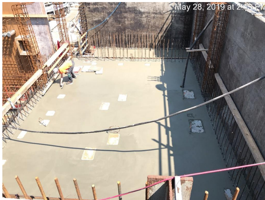
Figure 16 – Clover Point Pump Station – finishing suspended slab pour
