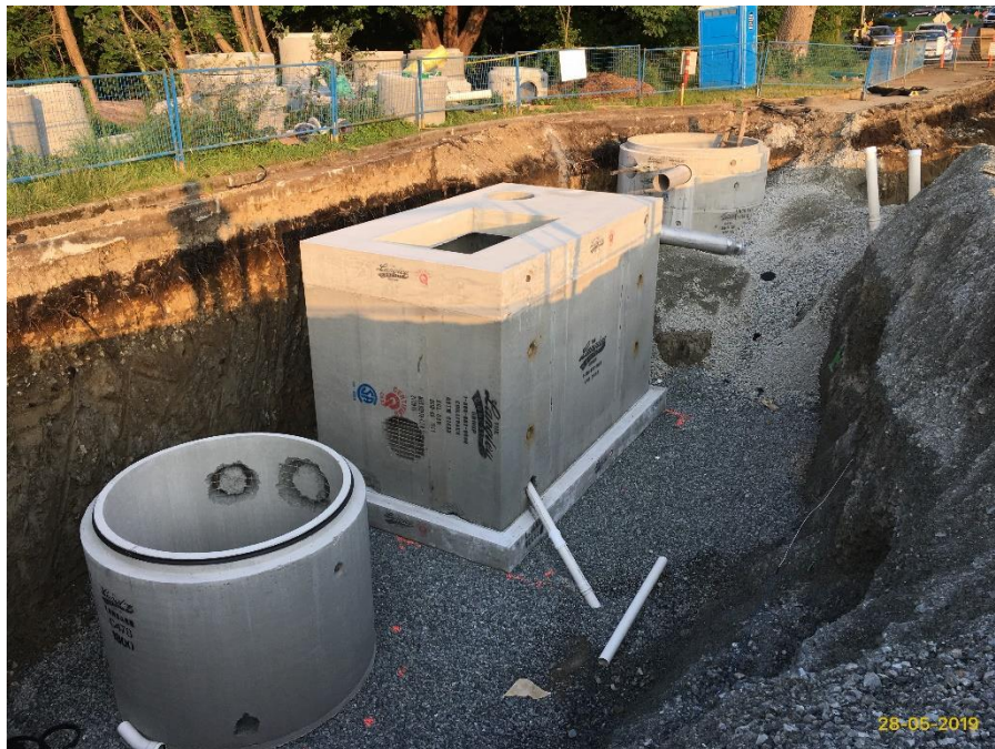
Figure 21 — Clover Forcemain: - installing odour control equipment east of Douglas Street.
