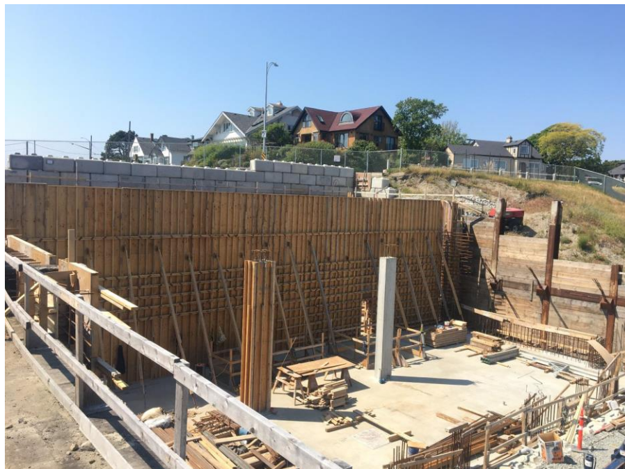
Figure 17 – Clover Point Pump Station – Site overview looking north west.
