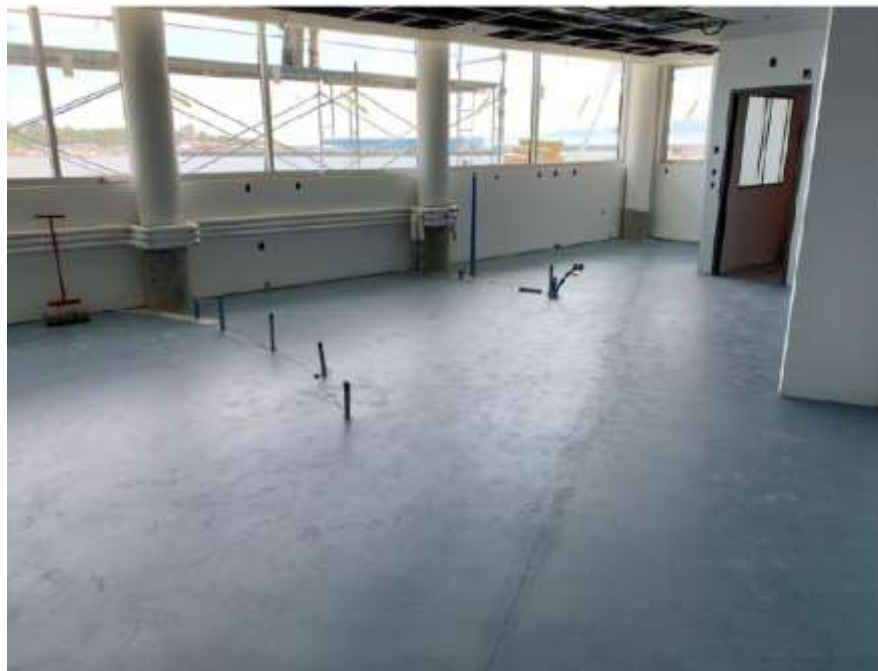
Figure 3– McLoughlin Point Wastewater Treatment Plant- Installed floor coating in the laboratory.
