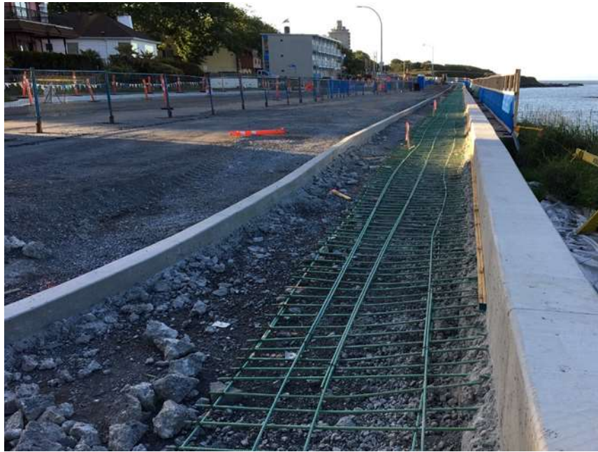
Figure 15–Clover Forcemain- New concrete wall replacing old balustrade wall, rebar installed for sidewalk and concrete curb delineating Cycle Track and sidewalk, Dallas Road from Dock Street looking east.
