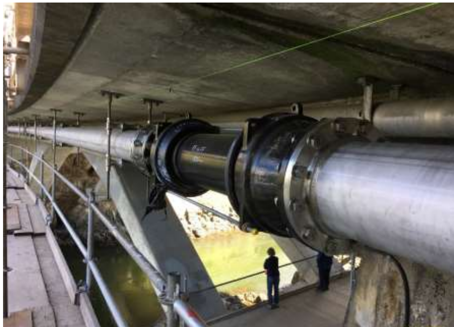
Figure 20 –Residual Solids Pump Stations – Tillicum Bridge pipe installed under Tillicum Bridge.
