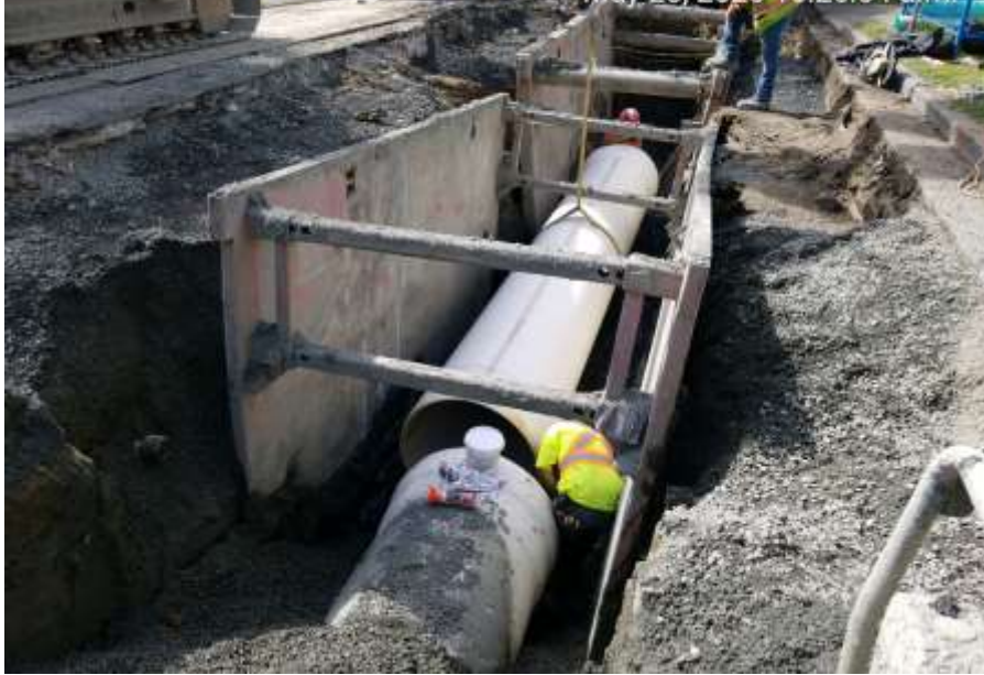
Figure 22- Trent Forcemain – Stannard Avenue – Forcemain installation progresses.
