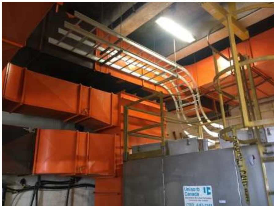
Figure 11- Clover Point Pump Station – Cable tray installation in screen & degritter room.
