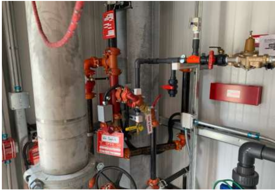
Figure 8- Residuals Treatment Facility – Fire protection water system mechanical installations nearing completion in Water Pump House.
