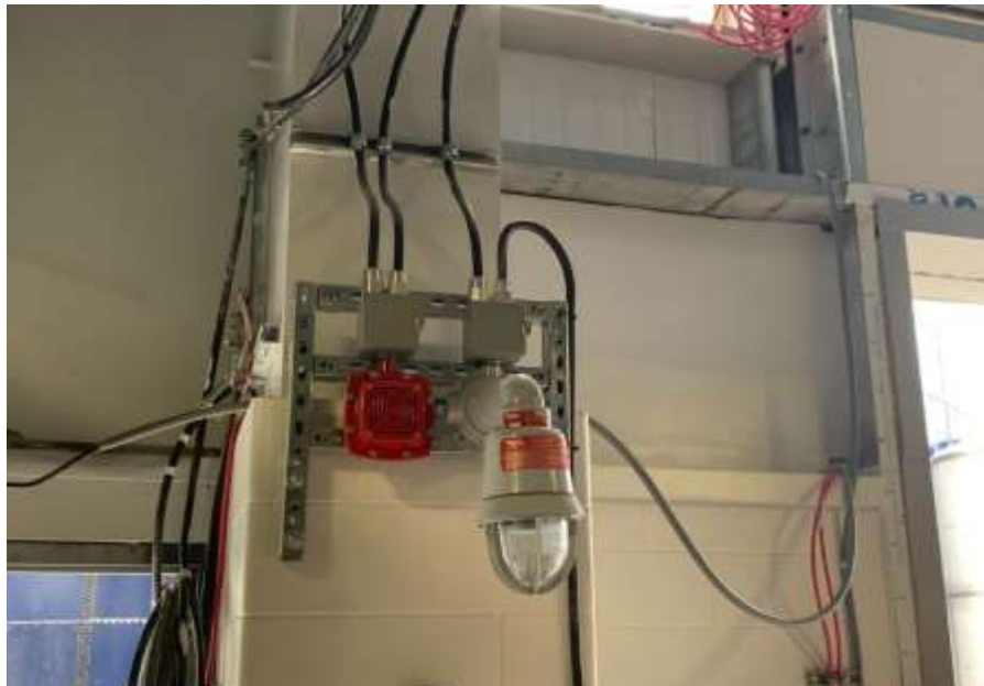
Figure 7- Residuals Treatment Facility- Installation of fire alarm systems ongoing throughout site.
