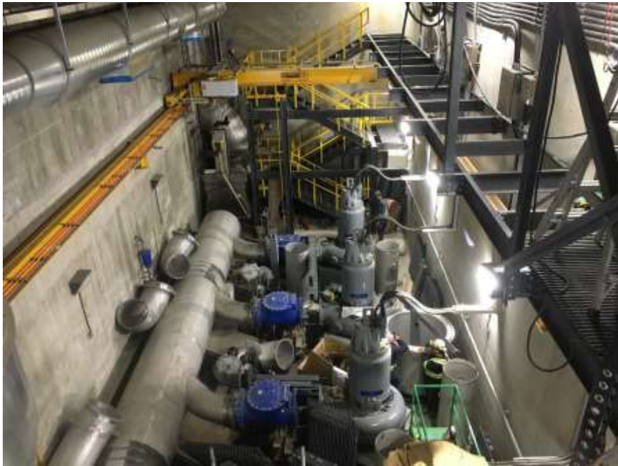
Figure 13-Macaulay Point Pump Station- Pump Room progression.
