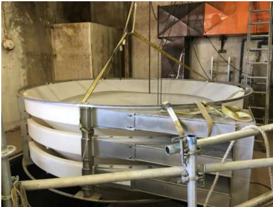
Figure 9–Clover Point Pump Station- Headcell installation.
