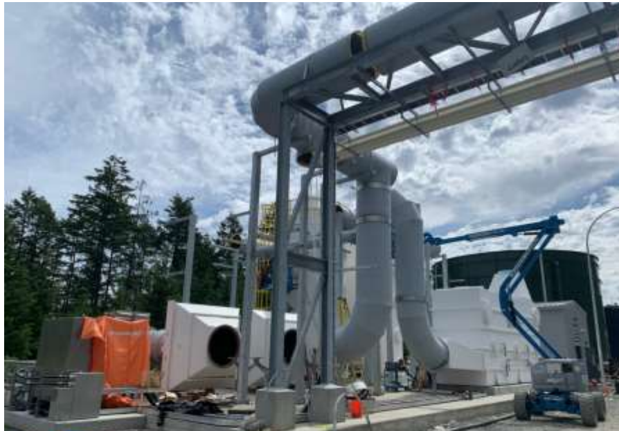
Figure 6- Residuals Treatment Facility- Installation of fiberglass reinforced plastic ducting for odour control systems being installed as well as structural supports.
