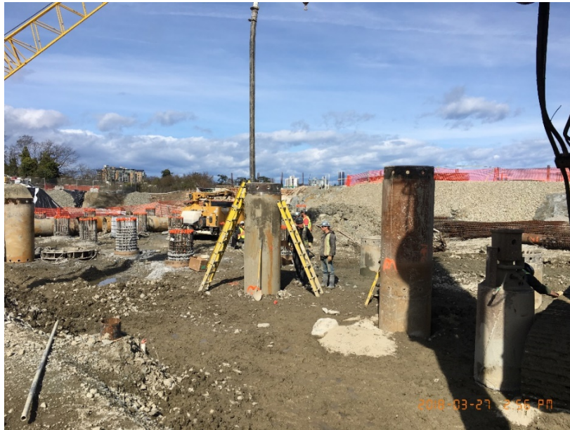
Figure 6 – Placing concrete in completed piles
