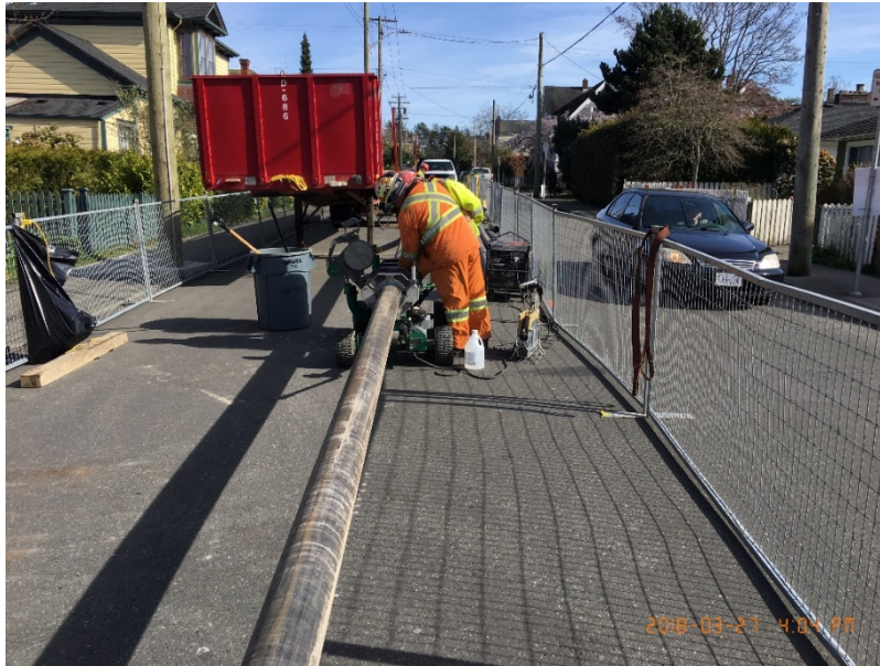
Figure 8 – Fusing of HDPE buoyancy pipe on Niagara Street
