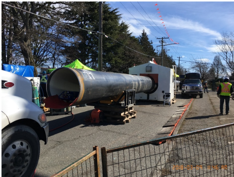
Figure 7 – Welding on Victoria Harbour Crossing pipe on Niagara Street
