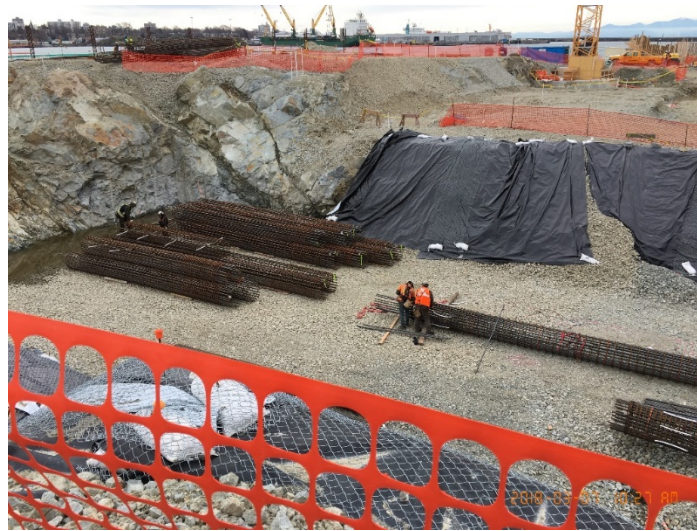
Figure 2 - Fabrication of rebar cages for piling
