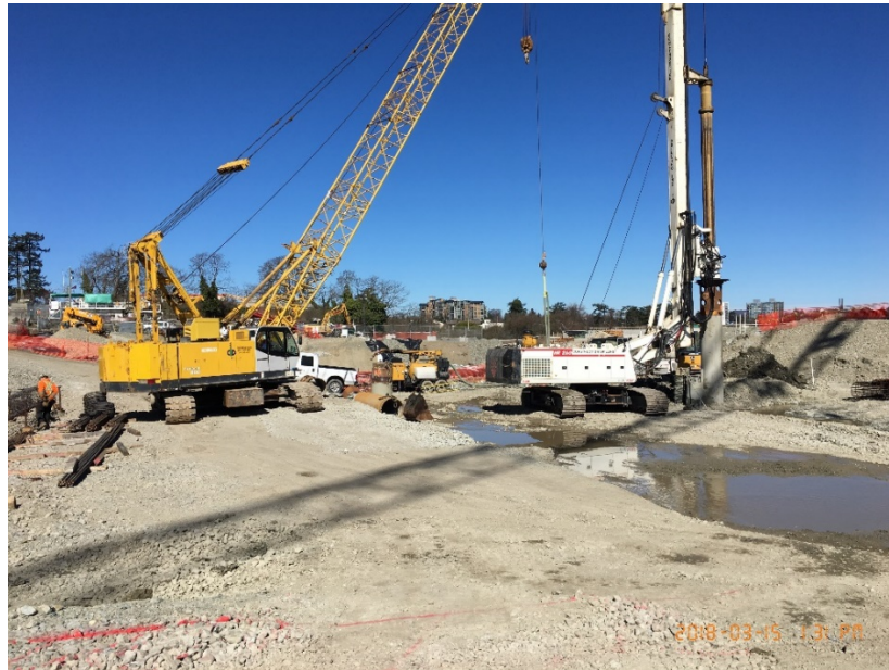
Figure 4 – Installing piles in the BAF area
