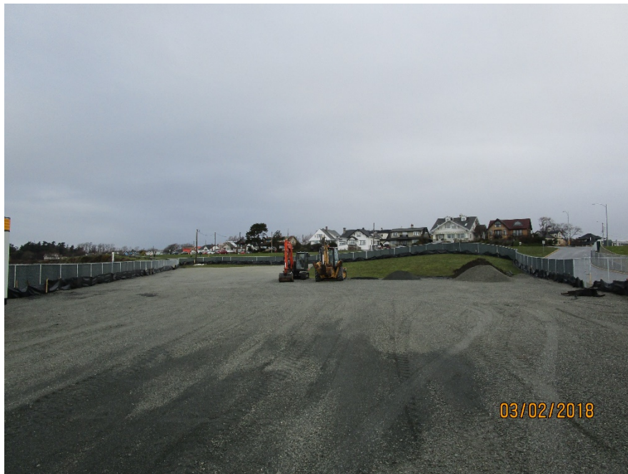
Figure 12 – View of west compound – Kenaidan's office compound and laydown area.
