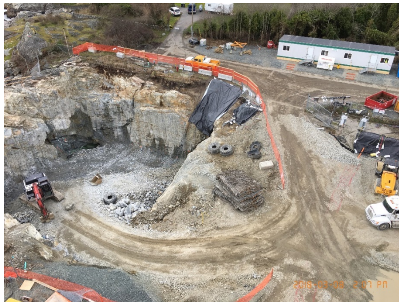
Figure 3 – Completed drilling, blasting and excavation of outfall shaft.
