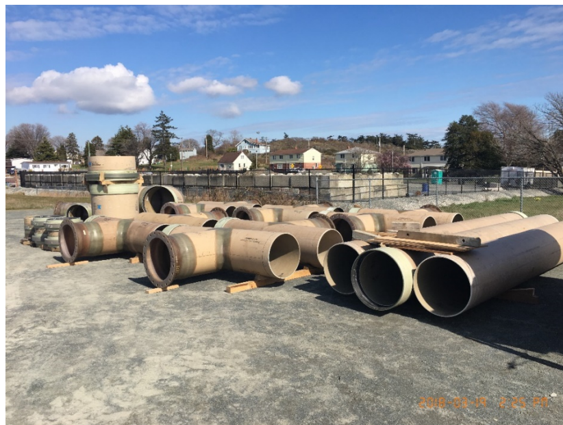
Figure 5 – Received Hobas pipe for BAF drainage
