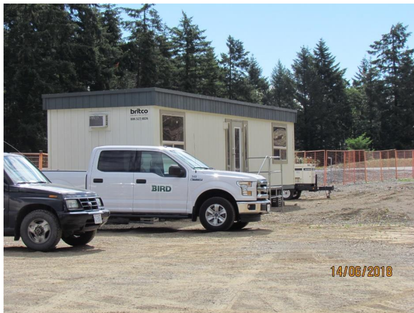
Figure 10 – Office trailer with temporary power connected.
