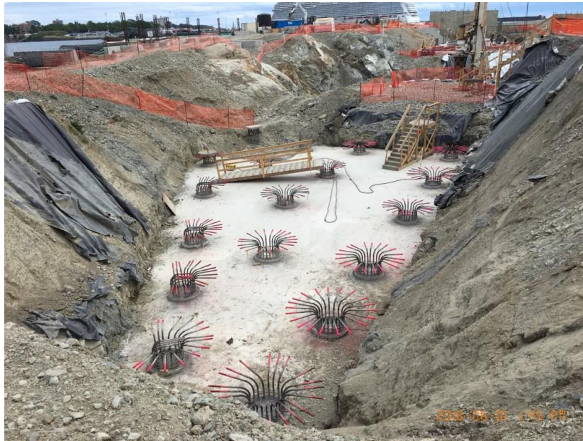
Figure 2 – Pile rebar bending complete in odour control area
