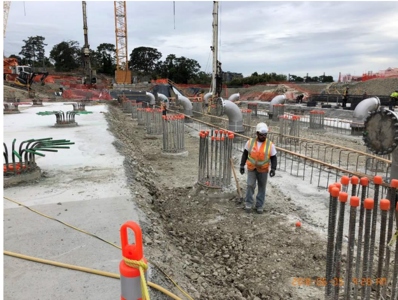
Figure 3 – Levelling of granular material in west biological aerated filters (BAF) gallery.
