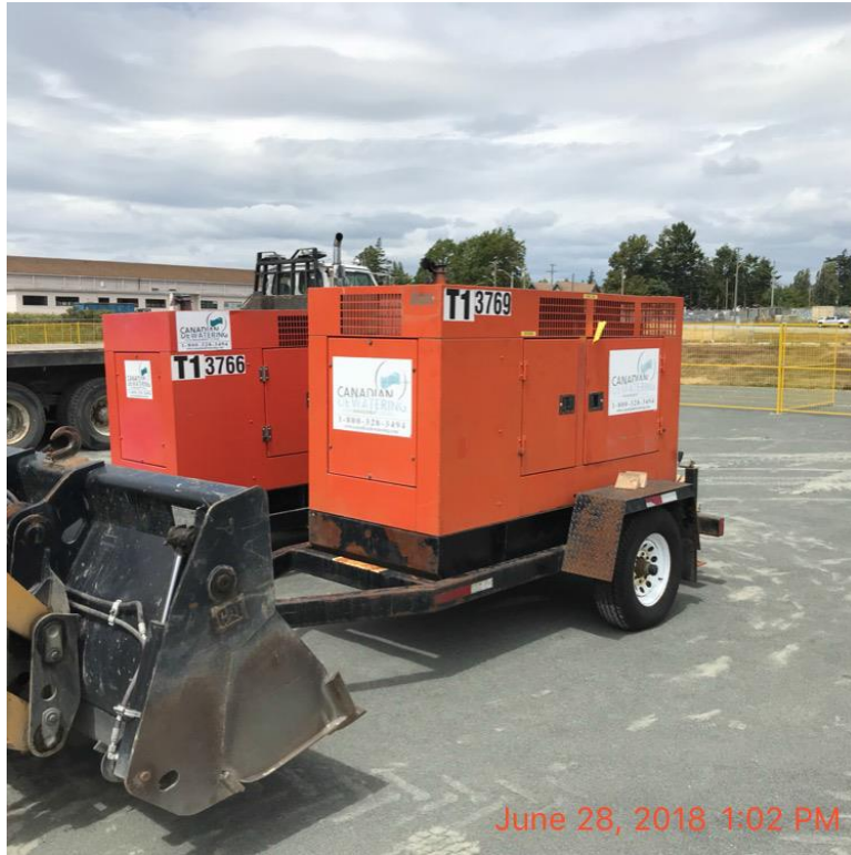
Figure 16 – pumps being set up for CCTV inspection
