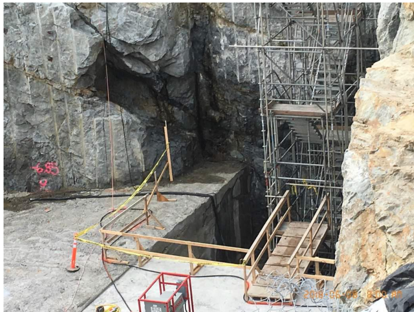
Figure 6 – Re-installing guardrail around outfall shaft.
