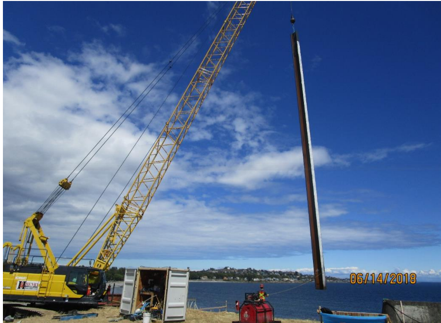
Figure 12 – Hoisting king pile #17 into place.
