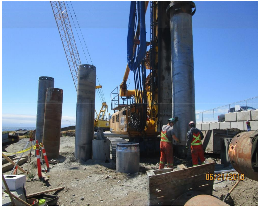
Figure 11 – Progressing king pile #20
