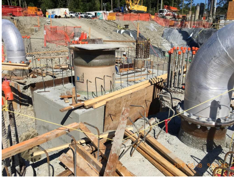
Figure 7 – Stripping forms from concrete pipe encasement.
