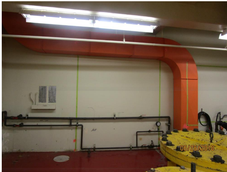
Figure 13 – Layout of future opening for new corridor and outfall pipe path at lower level.
