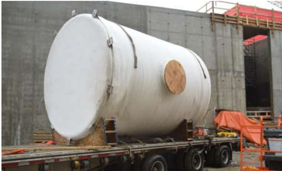
Figure 2– McLoughlin Point Wastewater Treatment Plant- Delivery of primary odour control tanks.
