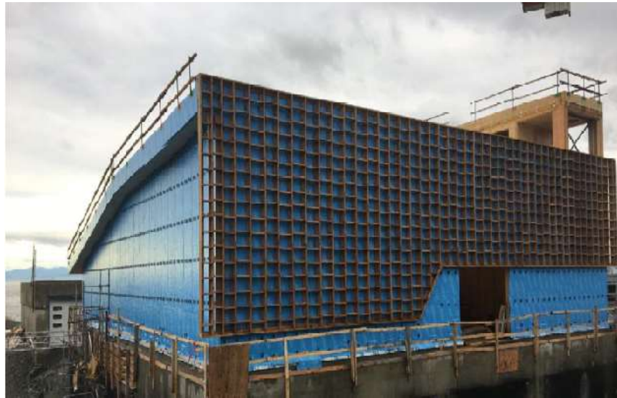
Figure 15–Macaulay Point Pump Station- CLT framing for architectural siding.
