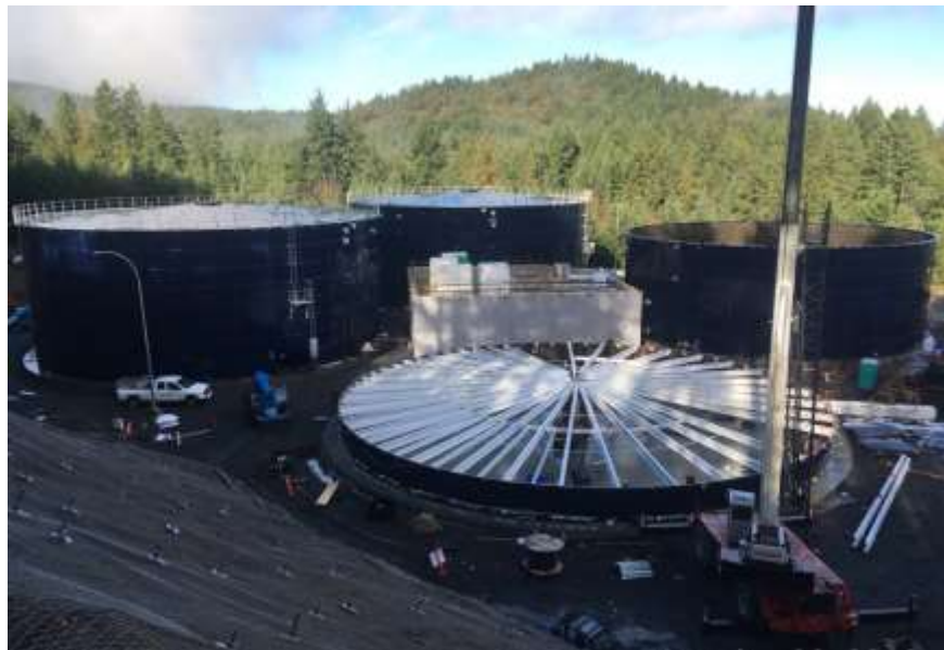
Figure 8– Residuals Treatment Facility- Digester 3 construction in progress.
