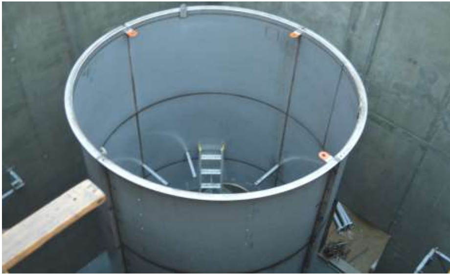
Figure 5- McLoughlin Point Wastewater Treatment Plant- Setting of Densadeg reactor tank.
