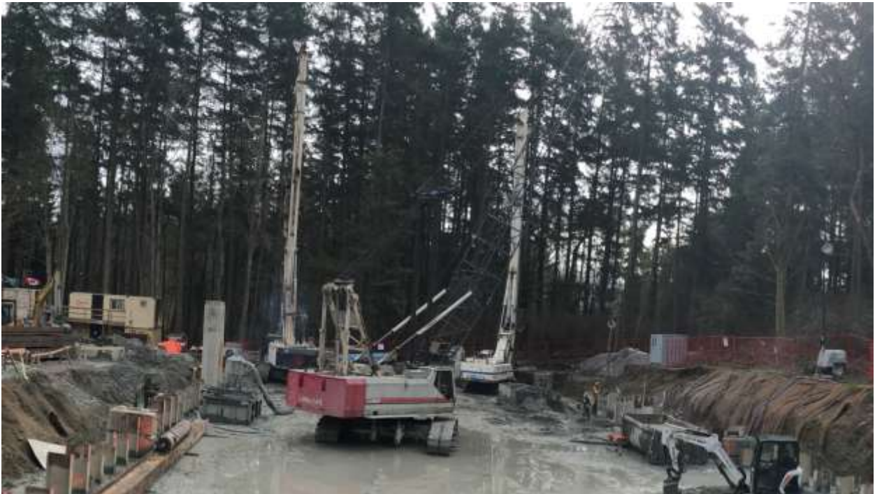
Figure 29– Arbutus Attenuation Tank –Ongoing piling w/ two drill rigs.
