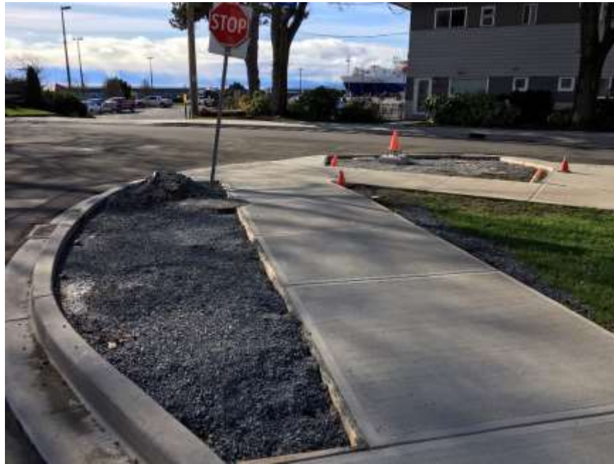
Figure 20–Clover Forcemain- Curb bump out and new sidewalk at Montreal Street.
