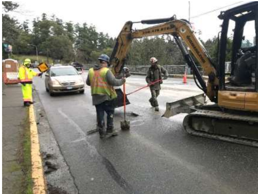
Figure 21–Residual Solids Pipes- Patching a pot hole on Tillicum Road.
