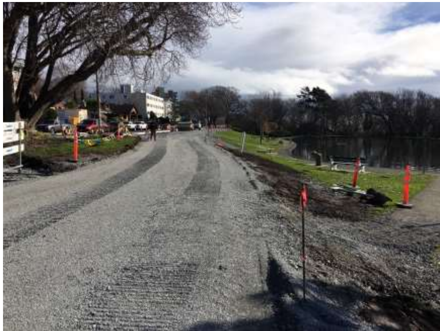
Figure 19–Clover Forcemain– Cycle track base preparation at Holland Park.
