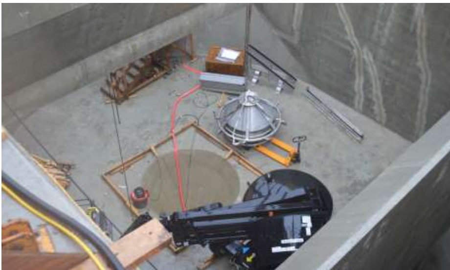
Figure 6- McLoughlin Point Wastewater Treatment Plant- Installing scraper cone in Densadeg 3 clarifier.
