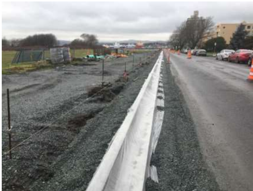
Figure 17–Clover Forcemain- Curb completed near South Turner Street.
