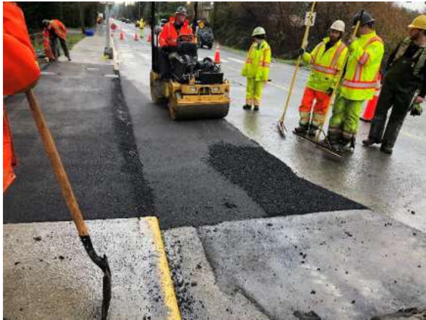
Figure 22–Residual Solids Pipes- Compaction of asphalt on Interurban Road.
