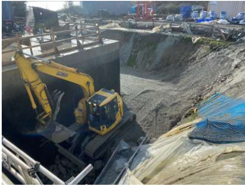
Figure 16–Macaulay Point Pump Station- Backfilling in the North West quadrant.
