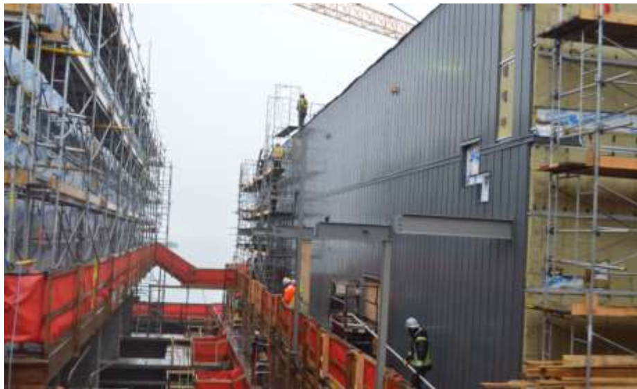
Figure 3- McLoughlin Point Wastewater Treatment Plant- Installing aluminium cladding.
