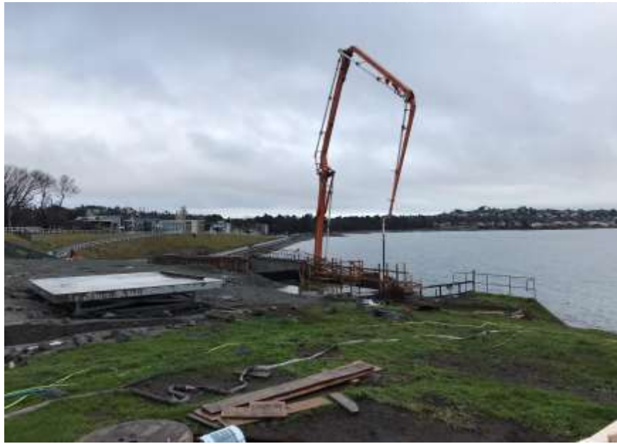
Figure 14- Clover Pump Station - South retaining wall concrete pour.
