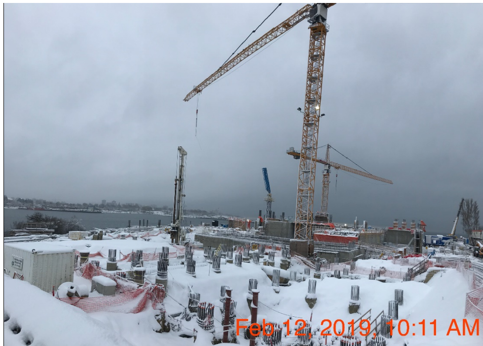
Figure 8 – McLoughlin Point Wastewater Treatment Plant: view looking south at snow-covered site.
