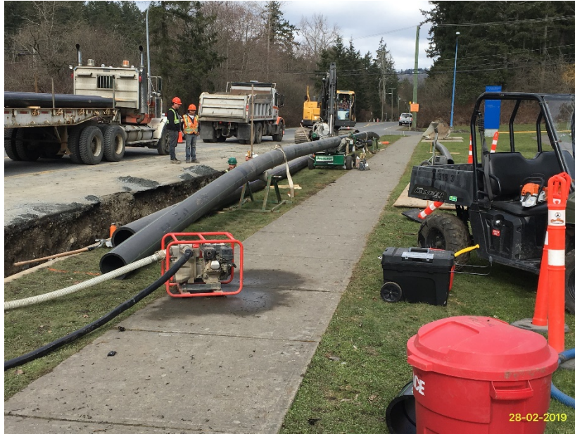
Figure 25 – RSCL: Segment 3 - installation of residual solids forcemain and centrate return line at Interurban Road.
