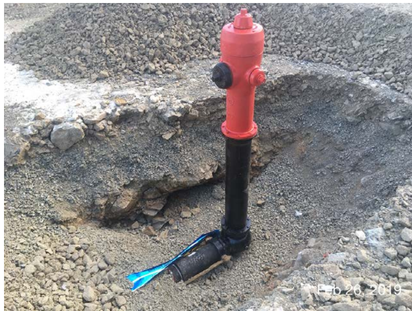
Figure 10 – Residuals Treatment Facility: installation of fire hydrants ongoing.
