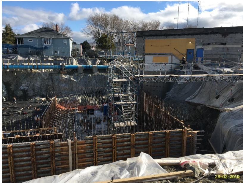
Figure 18 – Macaulay Point Pump Station: exterior wall formwork installed at west wall.
