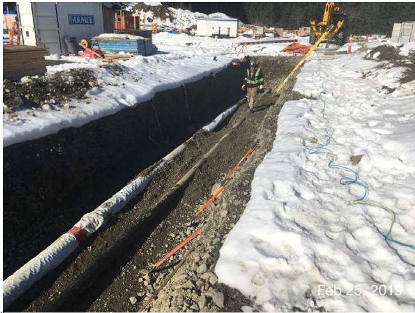
Figure 11 – Residuals Treatment Facility: backfilling process piping north of centrifuge building.
