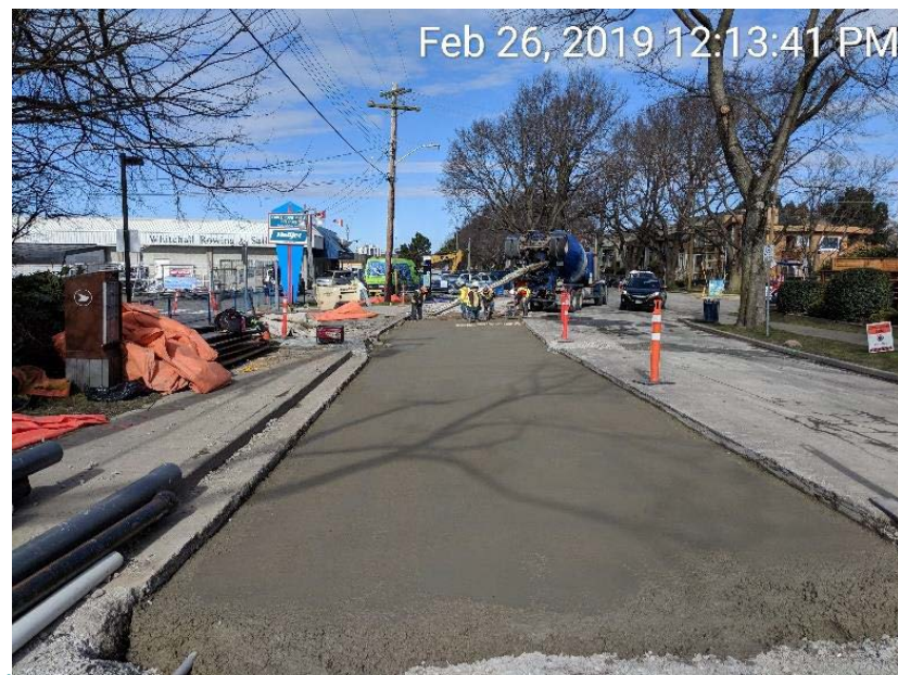
Figure 23 – Clover Forcemain: Dallas Road reinforced concrete cover slab complete.
