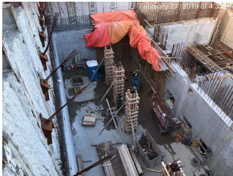
Figure 13 – Clover Point Pump Station: pump room column forms being completed.
