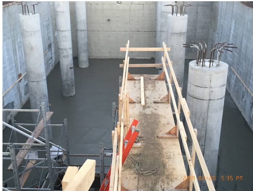
Figure 7 – McLoughlin Point Wastewater Treatment Plant: dirty backwash second topping pour.
