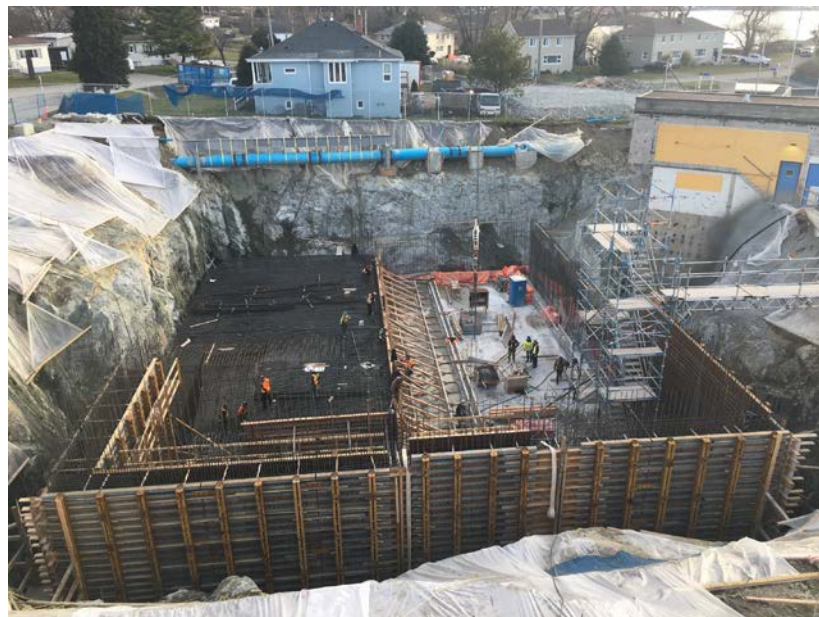
Figure 20 – Macaulay Point Pump Station: overview of pump station progression facing east.
