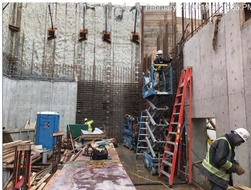
Figure 17 – Clover Point Pump Station: electrical conduit and form ties being installed.
