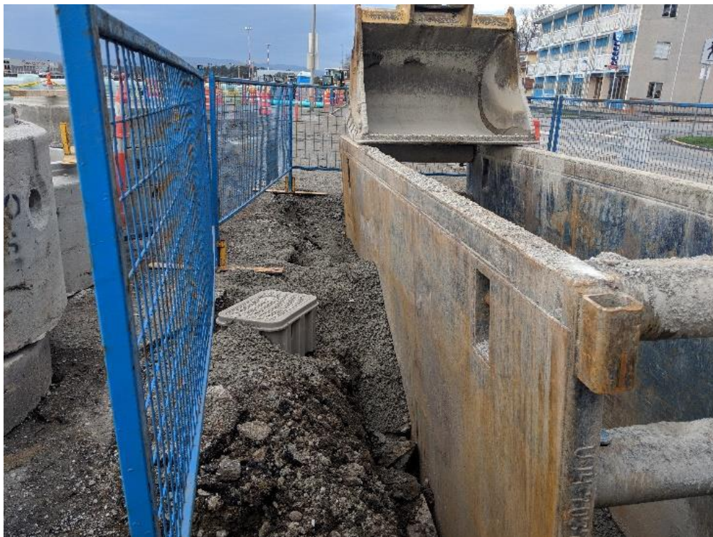
Figure 18 – Clover Forcemain: Dallas Road – trench shoring cage
