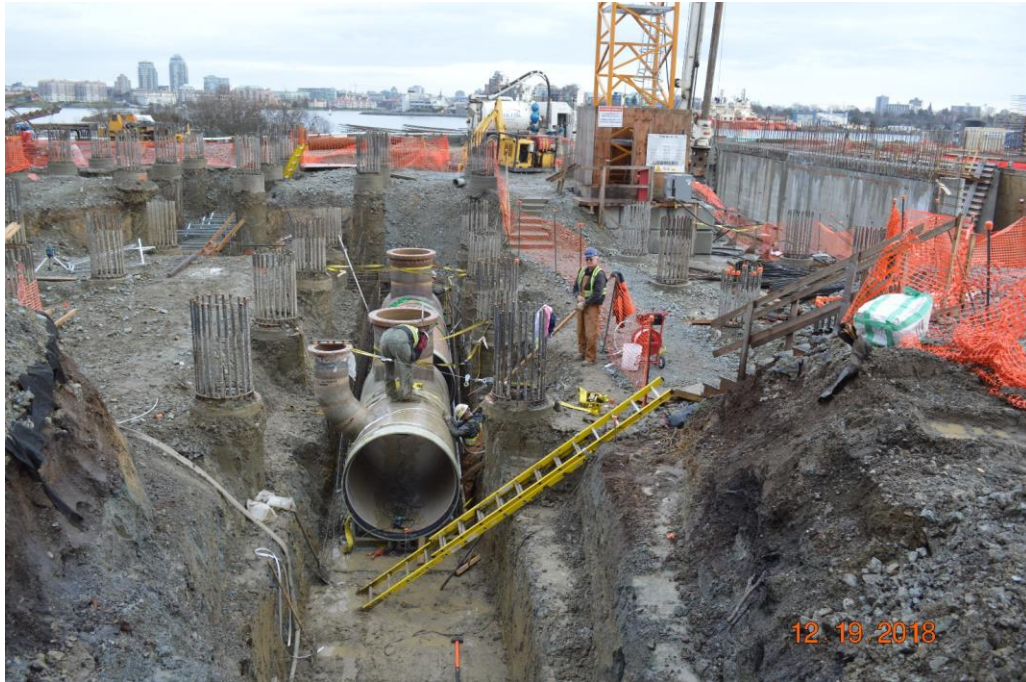
Figure 3 - McLoughlin Point Wastewater Treatment Plant: influent pipe placement in west Densadeg.
