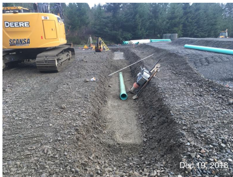
Figure 9 – Residuals Treatment Facility: installation of PVC drain main.
