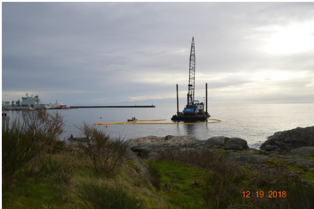
Figure 4 - McLoughlin Point Wastewater Treatment Plant: boom placement around outfall trenching barge.
