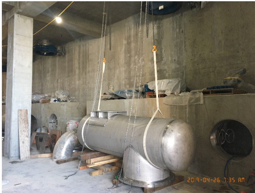
Figure 7 – McLoughlin Point Wastewater Treatment Plant: rigging 42" Header into position..
