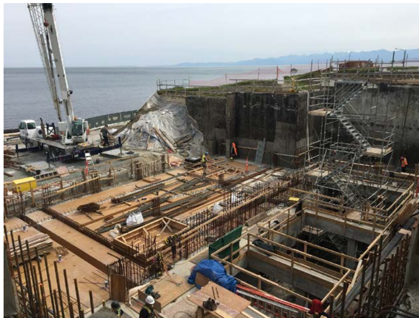
Figure 16 – Clover Point Pump Station general progress (view from north west).
