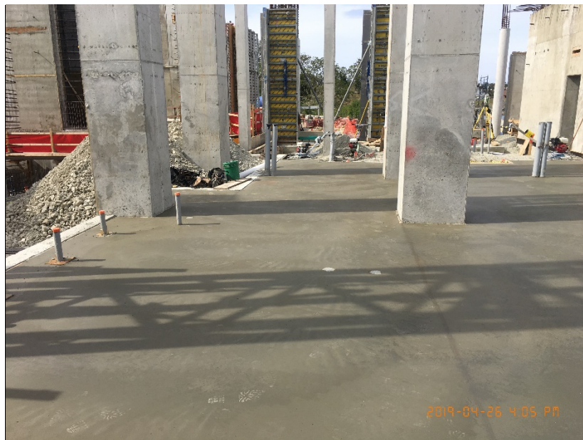
Figure 8 – McLoughlin Point Wastewater Treatment Plant: pouring slab.
