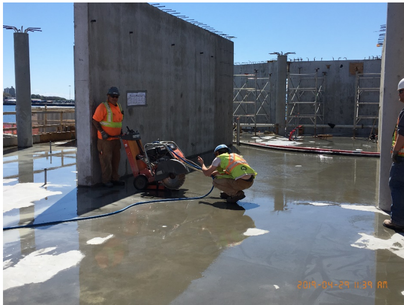
Figure 4 – McLoughlin Point Wastewater Treatment Plant: green cutting of control joints
