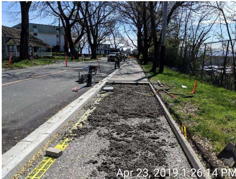
Figure 23 – Clover Forcemain: Dallas Road Island slip form placing concrete in sidewalks.
