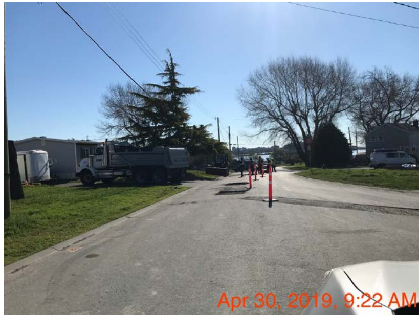
Figure 18 – Macaulay Point Forcemain digging test pits on Vaughan Street.
