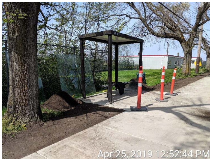
Figure 22 – Clover Forcemain: Bus shelter restored after sidewalk restoration
