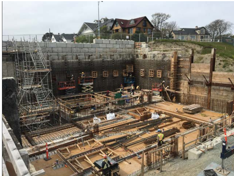
Figure 15 – Clover Point Pump Station: general progress (view from south east)
