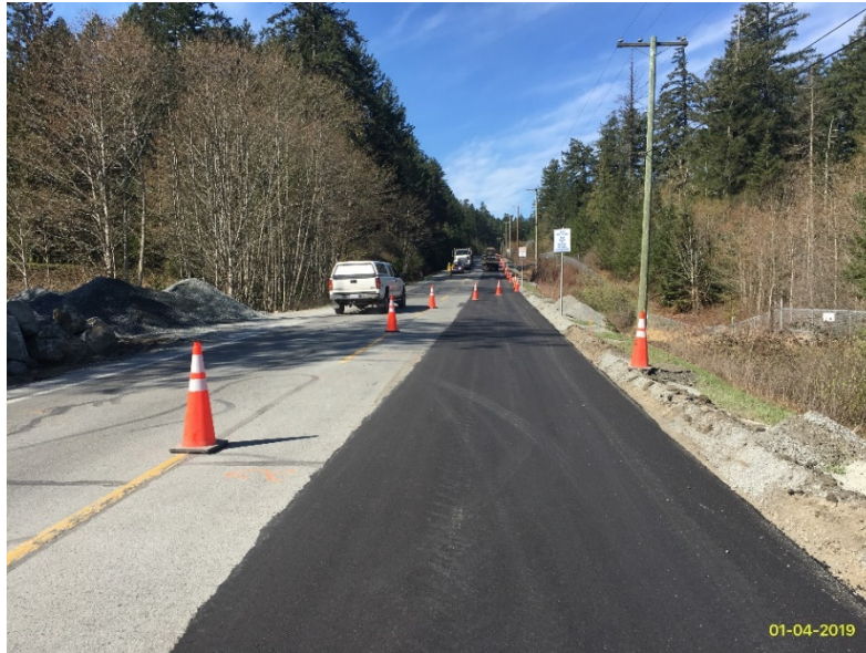
Figure 24 – RSCL: Segment 4 - installation of residual solids forcemain and centrate return line at Willis Point Road.
