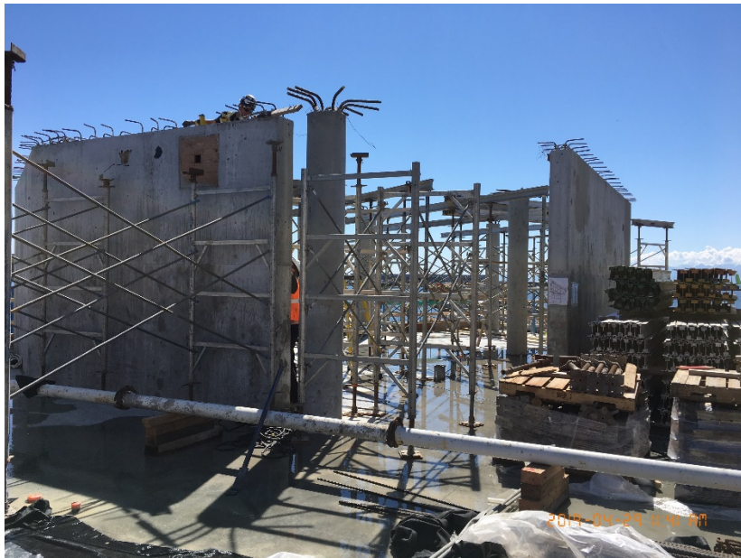
Figure 5 – McLoughlin Point Wastewater Treatment Plant: installing scaffolding for suspended slab #1.
