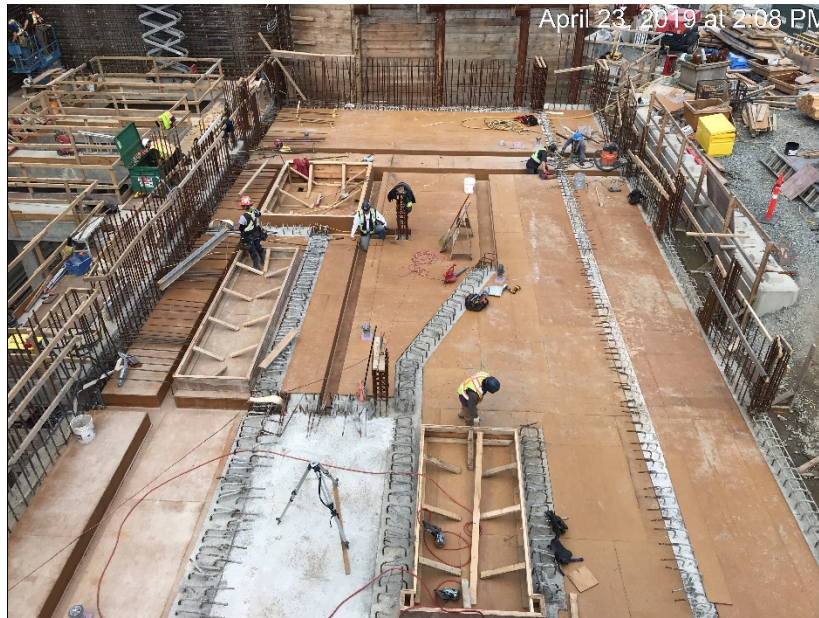
Figure 17 – Clover Point Pump Station: installing formwork for suspended slab.
