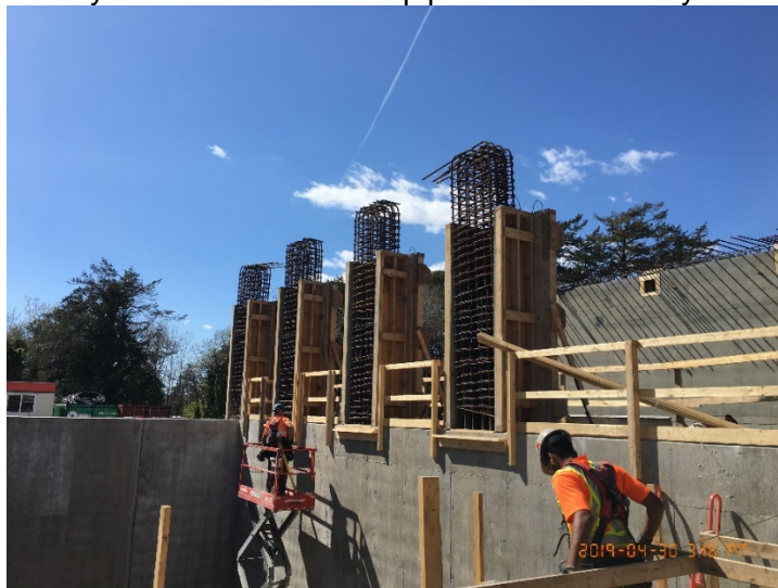
Figure 2 – McLoughlin Point Wastewater Treatment Plant: Forming BAF wall 10 columns
