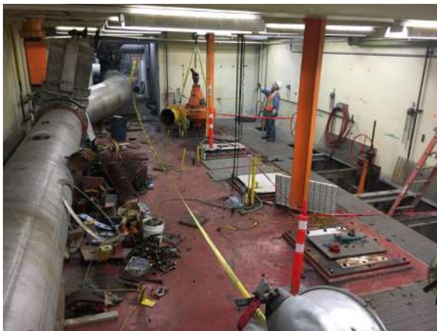
Figure 13- Clover Point Pump Station – Demolition of room.
