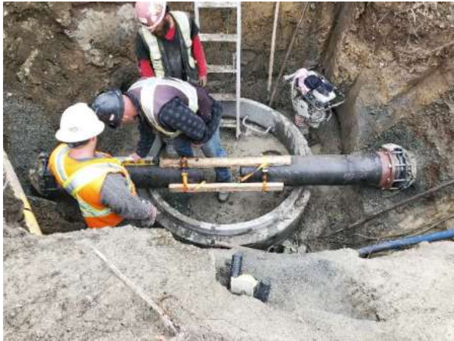
Figure 20–Residual Solids Pipes – Aligning pipe for line valve on Colquitz Road.
