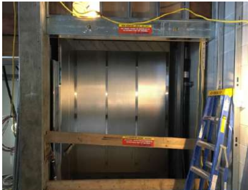
Figure 2– McLoughlin Point Wastewater Treatment Plant - Installing elevator cab.
