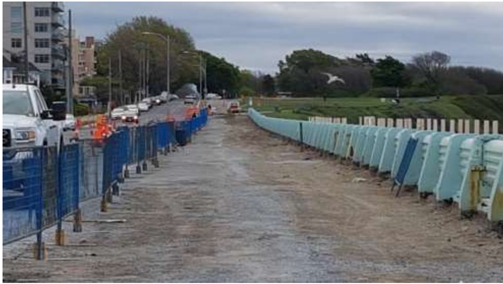
Figure 17–Clover Forcemain- Seawall balustrade construction set up.
