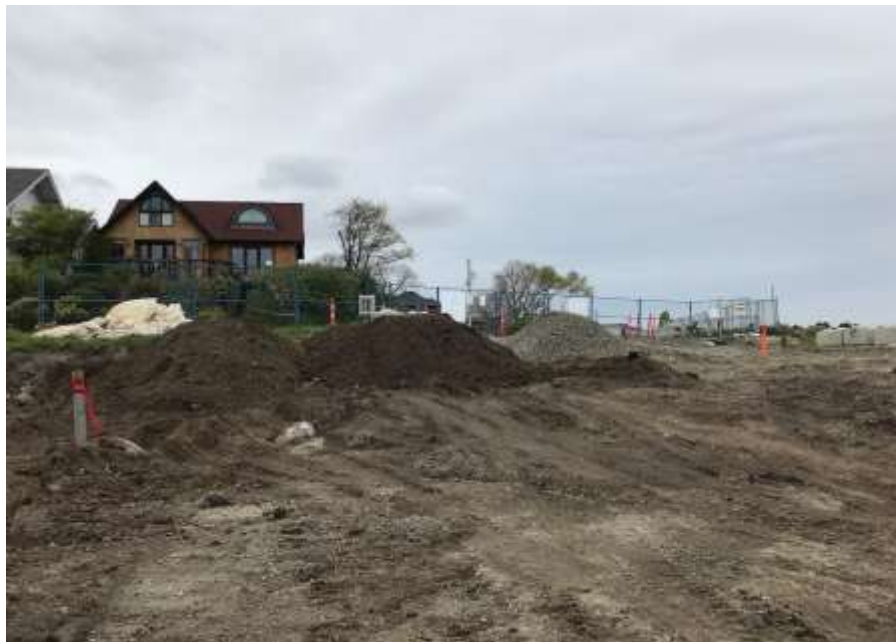
Figure 12-Clover Point Pump Station- Backfilling of the forcemain ongoing.
