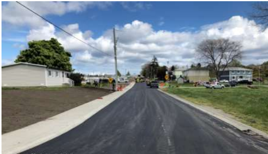
Figure 14–Macaulay Point Pump Station- Base course of asphalt on Anson Street.
