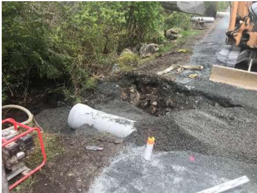
Figure 21–Residual Solids Pipes - Installing culvert across Interurban Trail.
