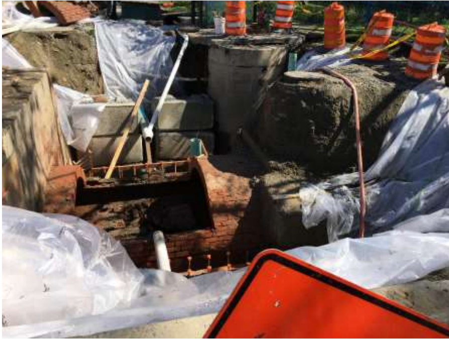
Figure 25- Trent Forcemain – Bushby Street – excavate and demolish existing brick drain.
