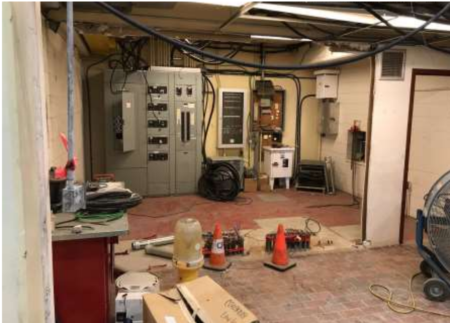
Figure 11–Clover Point Pump Station- Electrical equipment demolition in the old electrical room.
