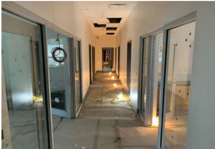
Figure 10– Residuals Treatment Facility – Interior finishing of Operations Building ongoing.
