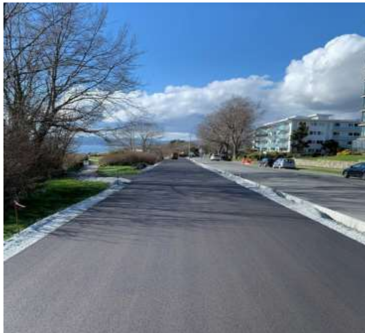
Figure 16–Clover Forcemain- Cycle track/road restoration from Government Street to Lewis Street.
