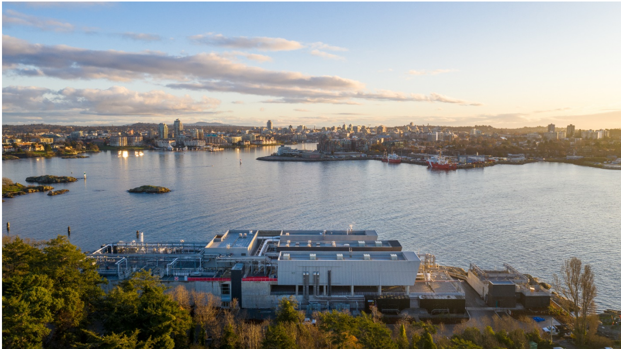
Figure 2 – Looking east over the McLoughlin Point Wastewater Treatment Plant
