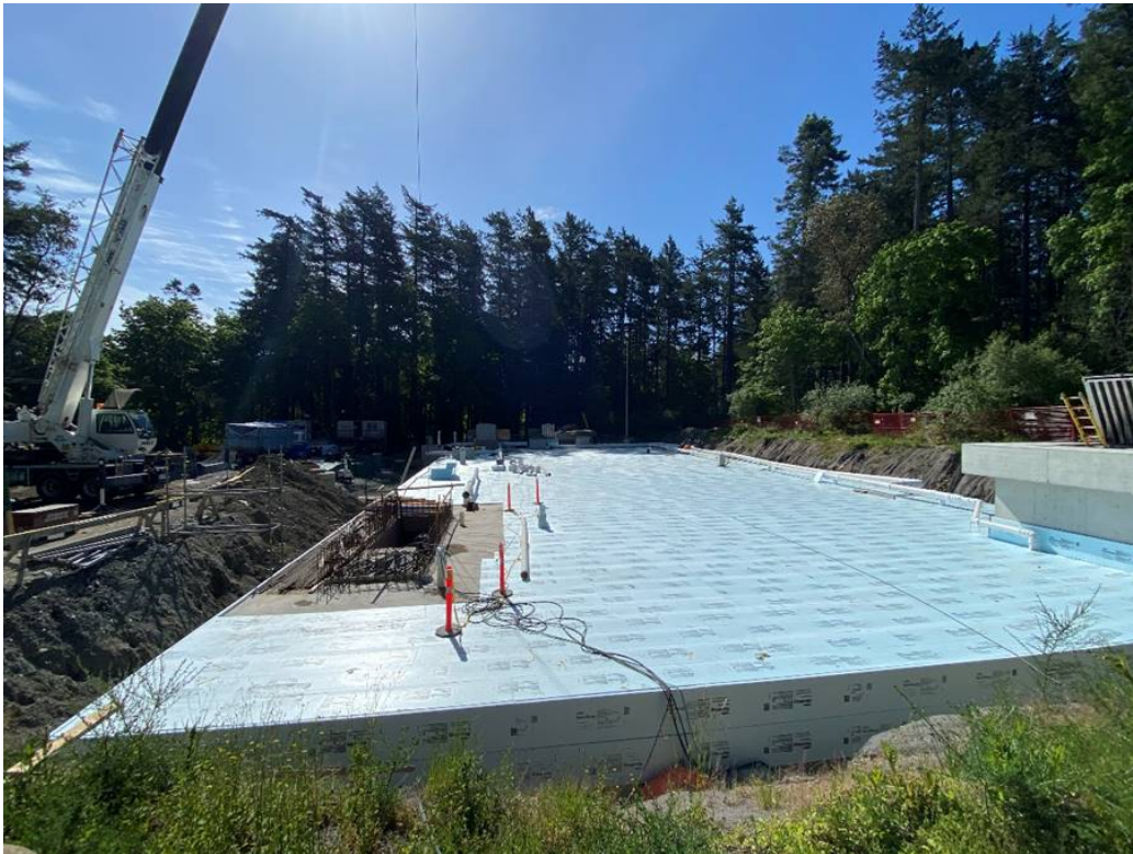
Figure 14 – Arbutus Attenuation Tank (Construction in progress)
