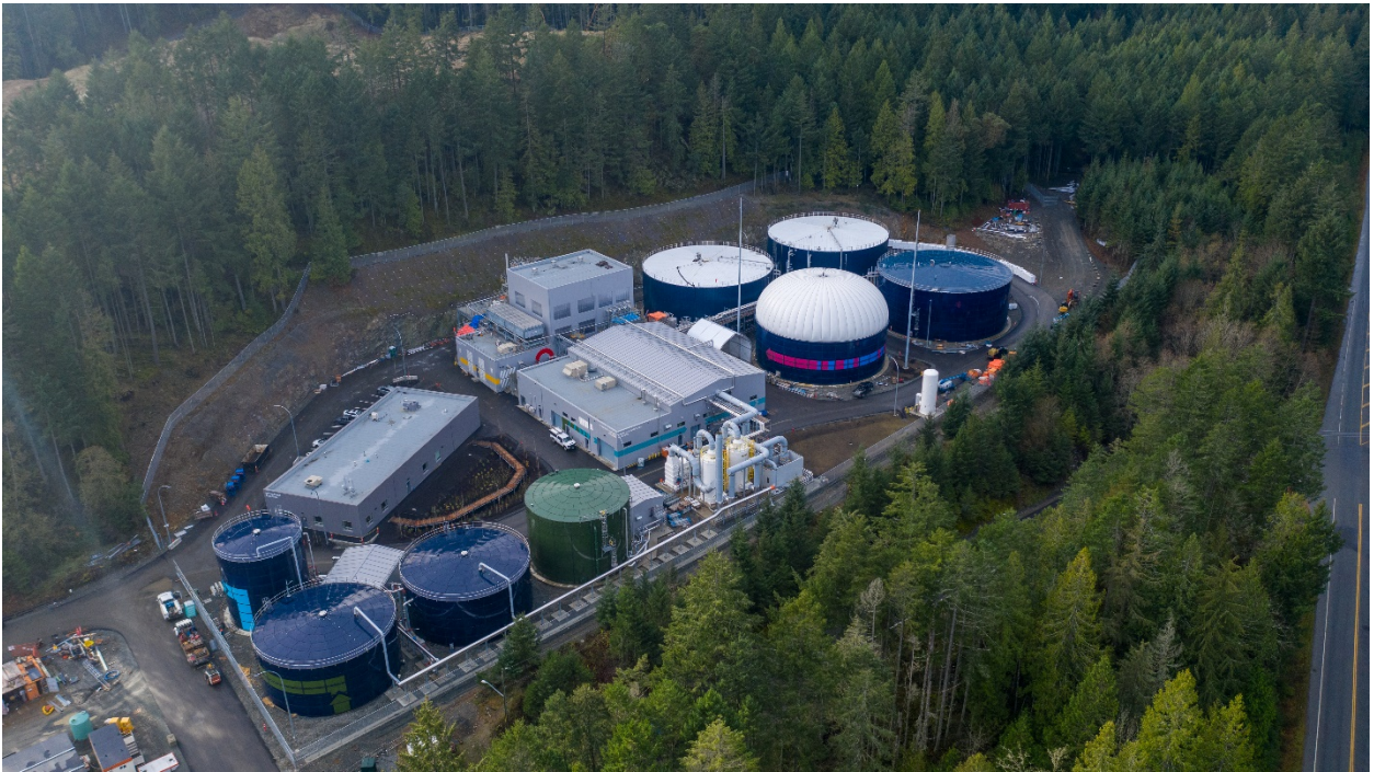
Figure 3 – Looking southwest toward the Residuals Treatment Facility
