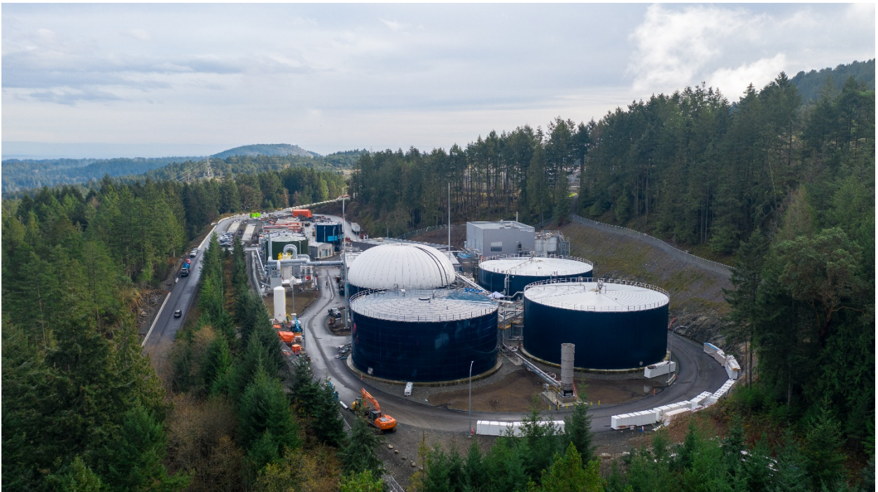
Figure 4 – Looking east toward the Residuals Treatment Facility
