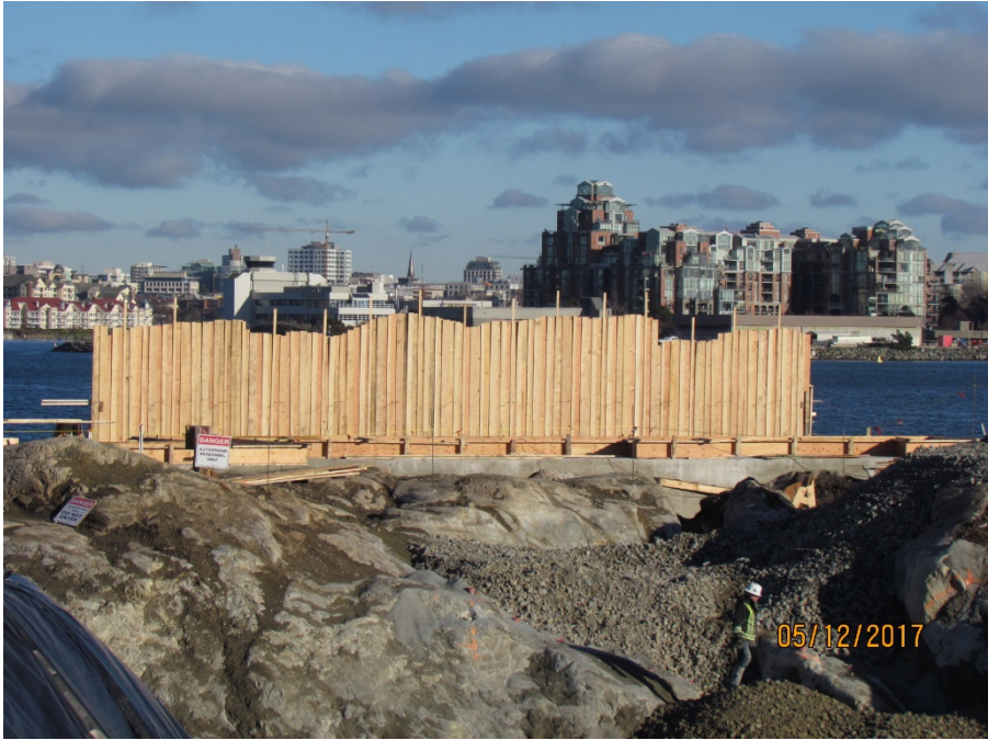
Figure 3 – Planter wall vertical board forms
