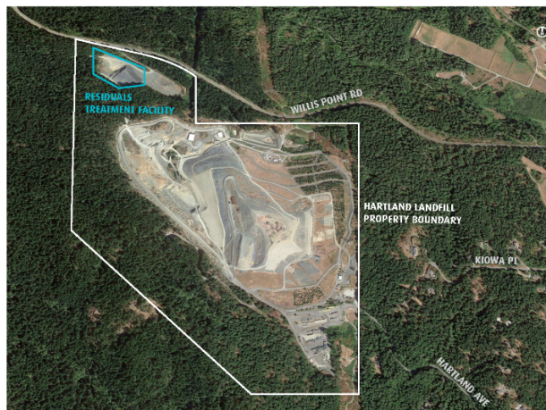
Residuals Treatment Facility site within the Hartland Landfill
