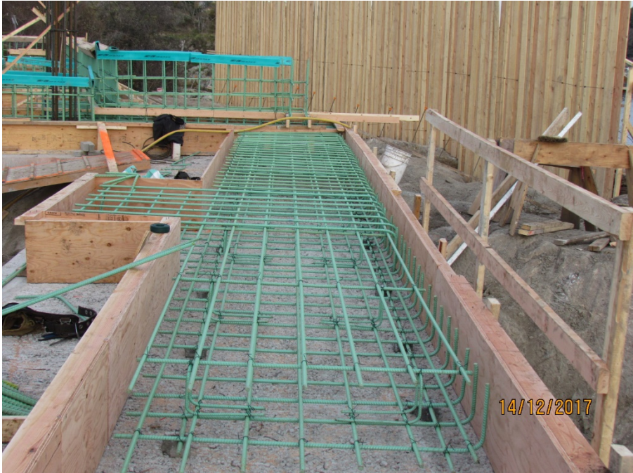
Figure 2 - Tsunami wall footing formed with epoxy coated rebar
