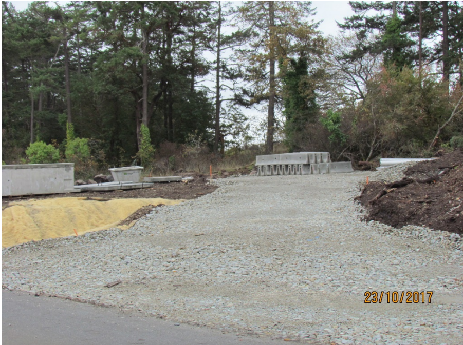
Figure 5 – Construction of truck turnaround on Victoria View Road
