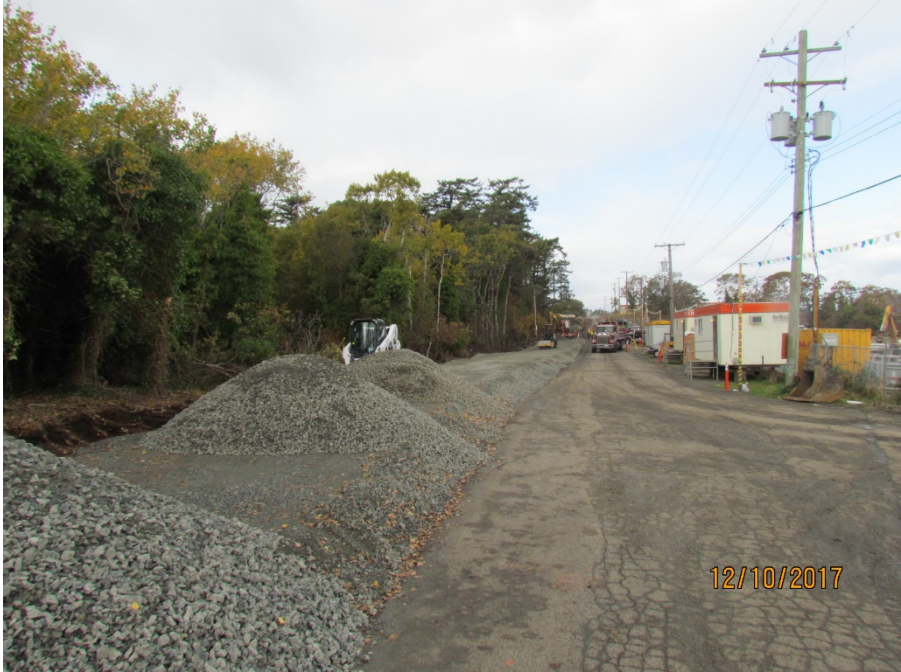
Figure 6 – Road widening & BC Hydro Right of Way on Victoria View Road
