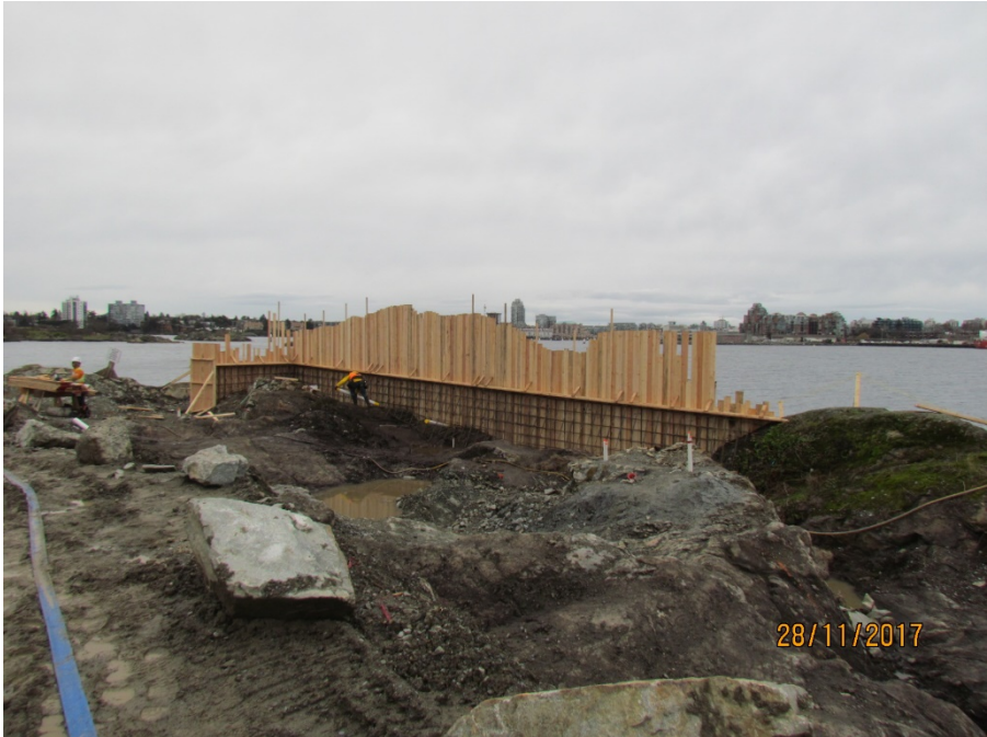
Figure 7 – Planter wall board forms with rebar installed
