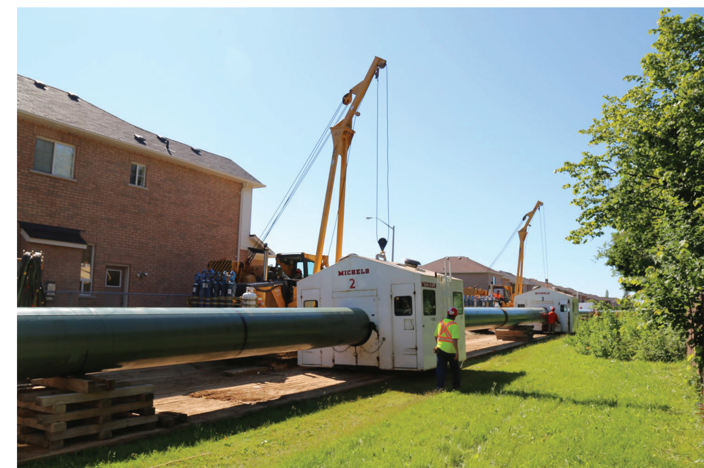
Example of a welding enclosure
