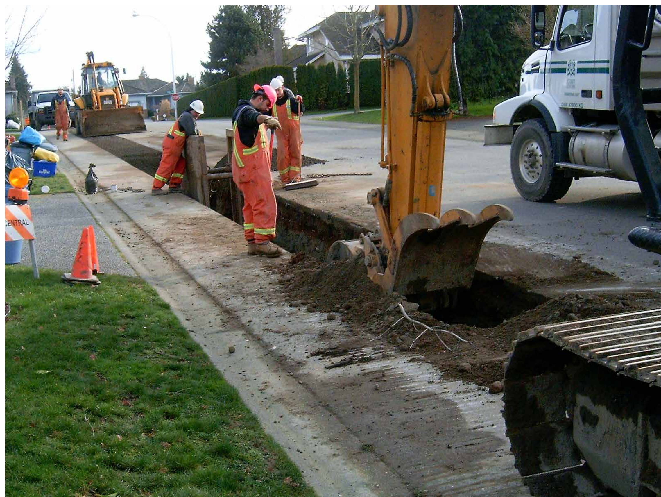
Example of pipe installation
