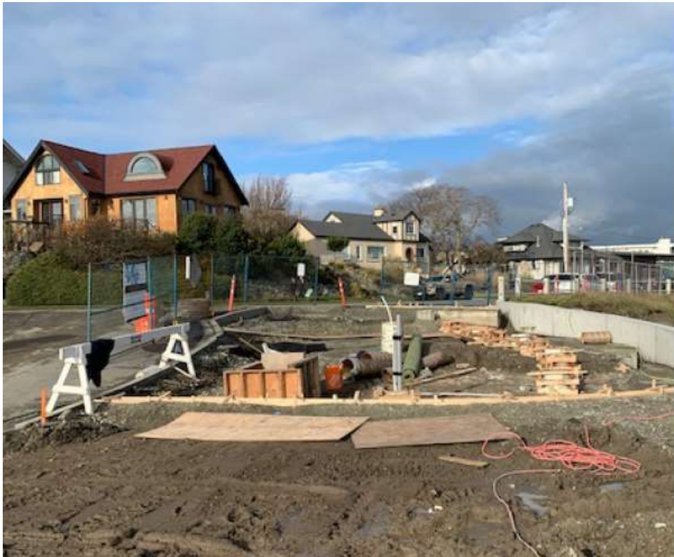
Figure 6 – Clover Point Pump Station - Conduit area preparation.
