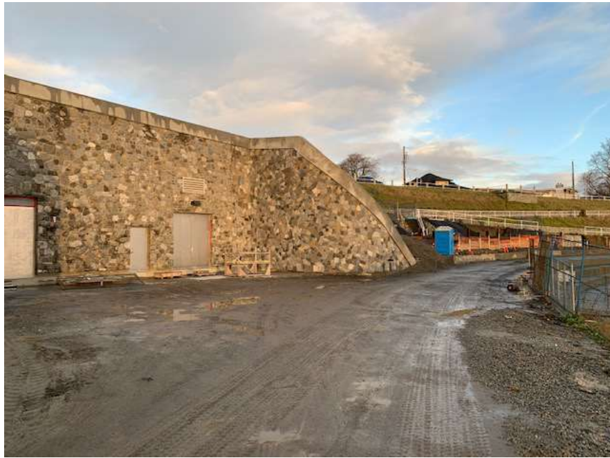
Figure 7 – Clover Point Pump Station - Rock face on new pump station.
