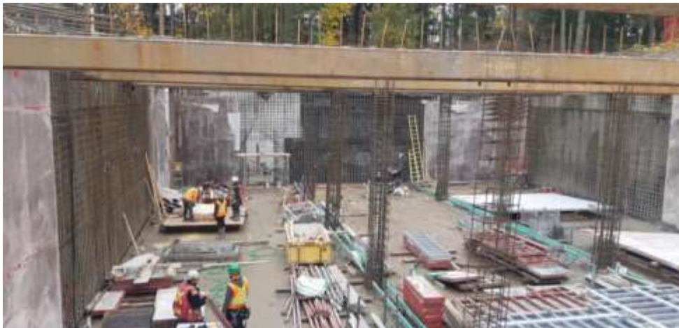
Figure 12 – Arbutus Attenuation Tank- Column reinforcing installation process.
