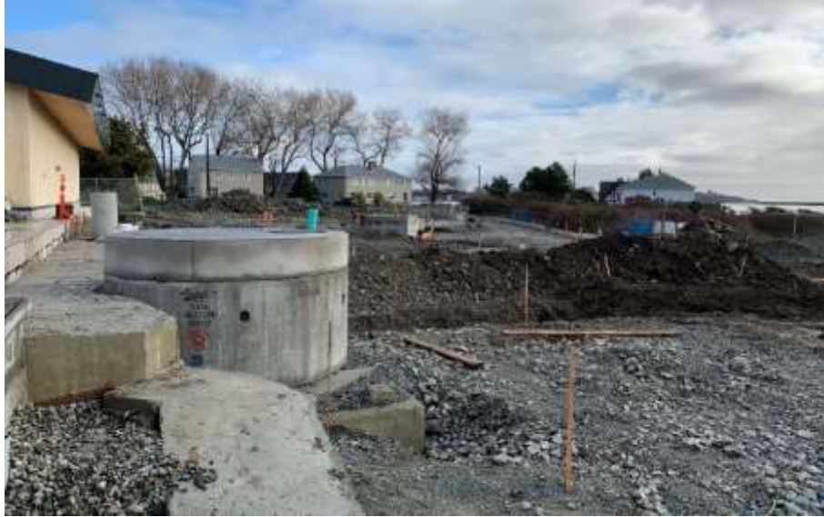
Figure 8 – Macaulay Point Pump Station - Demolition of old Pump Station completed
