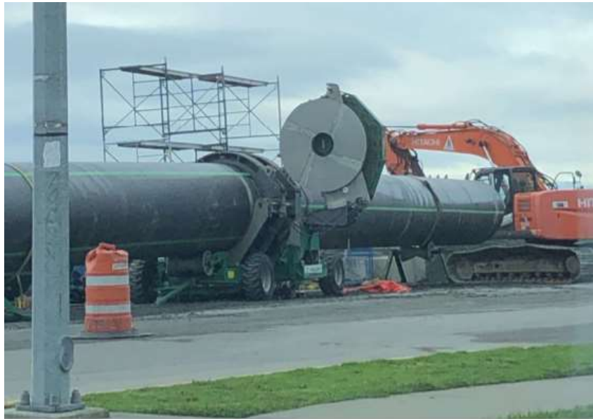
Figure 14 – Trent Forcemain - Fusion of High Density Polyethylene Pipe.
