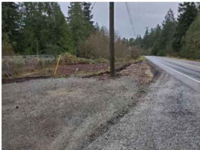
Figure 11 –Residual Solids Pump Stations – Restoration of Willis Point Road Laydown area.
