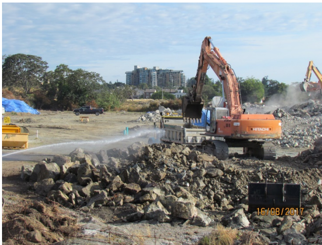
Figure 5 – Loading blast rock on to trucks and hauling to area A
