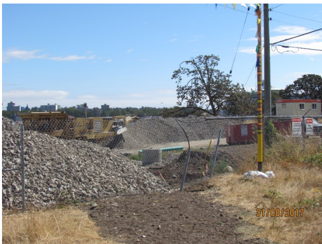
Figure 6 – Crushed blast rock in area A
