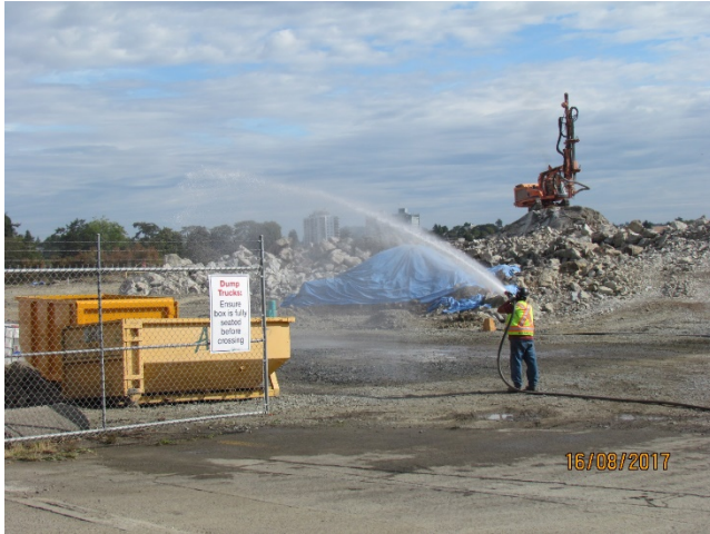
Figure 4 - Maintaining dust control on site
