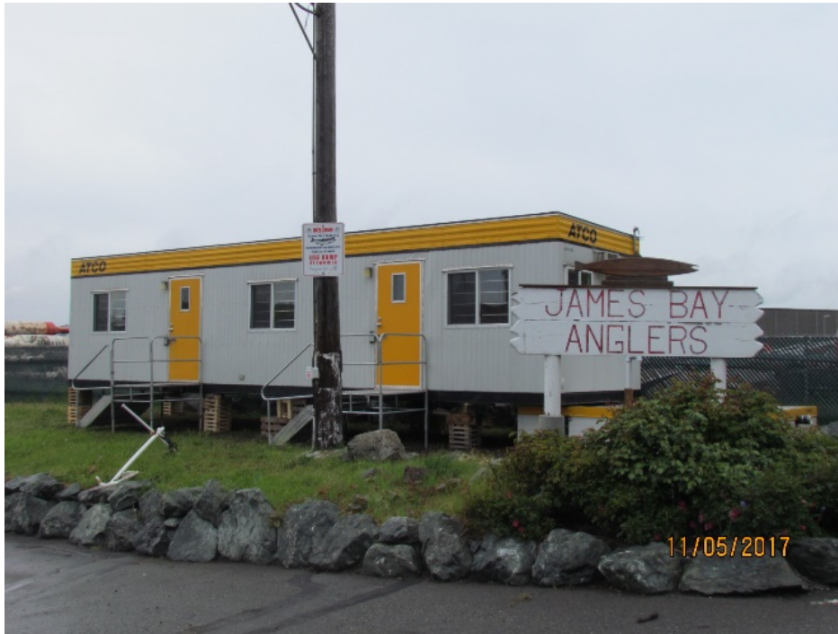
Figure 3- Temporary Angler's Hut delivered and set up
