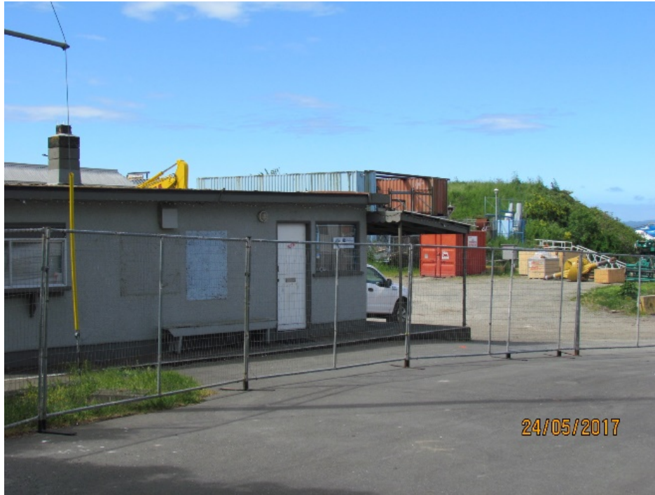
Figure 5- Temporary fencing installed
