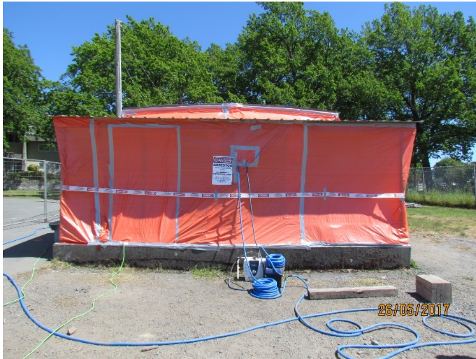
Figure 2- Negative air pressure asbestos enclosure
