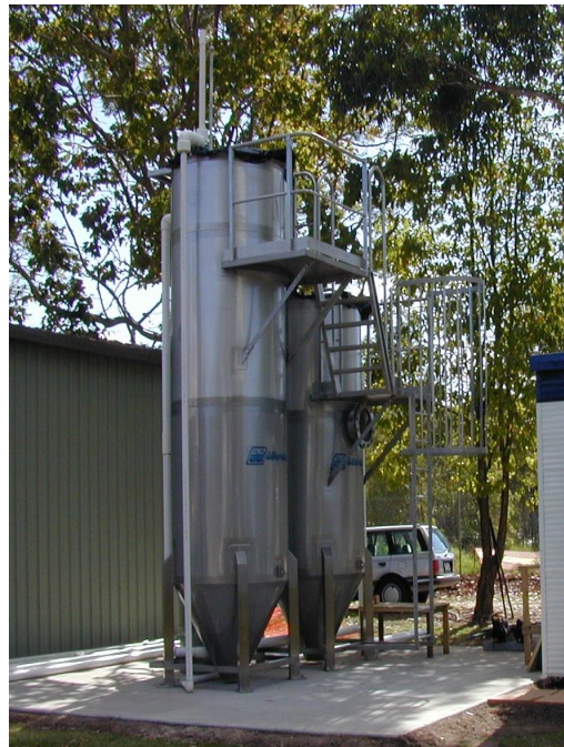
A CleanStream™ 950 m 3 /d module
