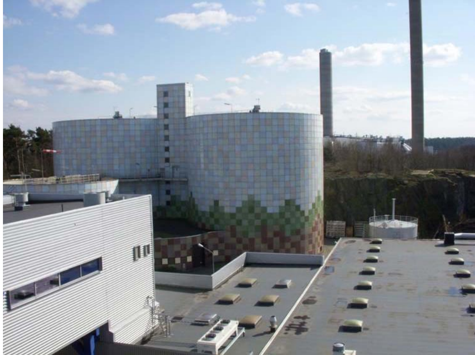
Figure 6 The Anaerobic Digesters at the Gryaab WWTP
