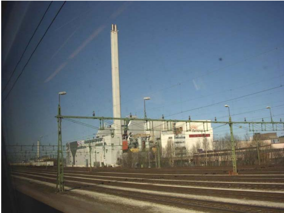
Figure 1 The Renova MSW WTE Facility (Note the lack of visible plume from the stack)
