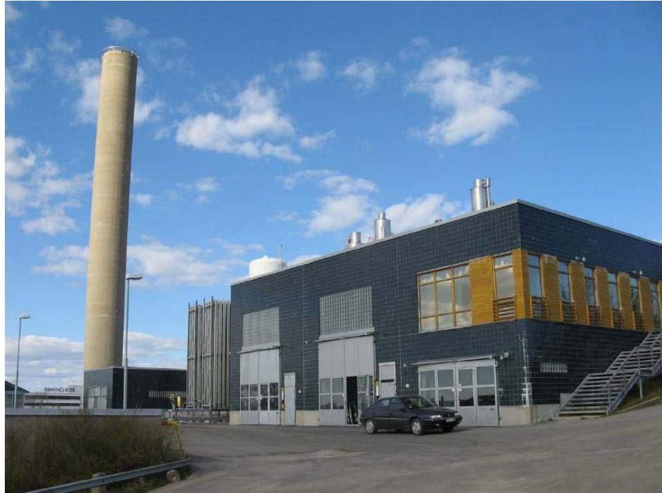
Figure 10 The Biogas Upgrading Facility at the Henriksdal Reningsverk (Stack at left is part of the plant odour control system, not related to the biogas upgrading facility)
