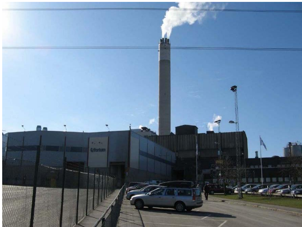
Figure 3 Fortum Energi Högdalen MSW WTE Facility in Southwest Stockholm
