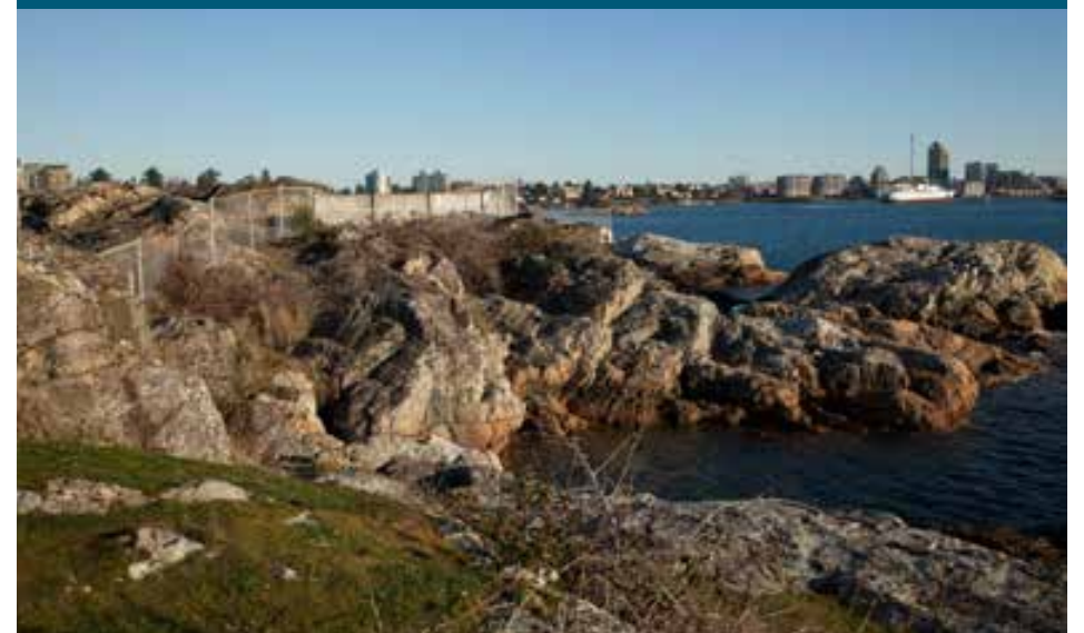
>> Site of the Treatment Plant at McLoughlin Point.
