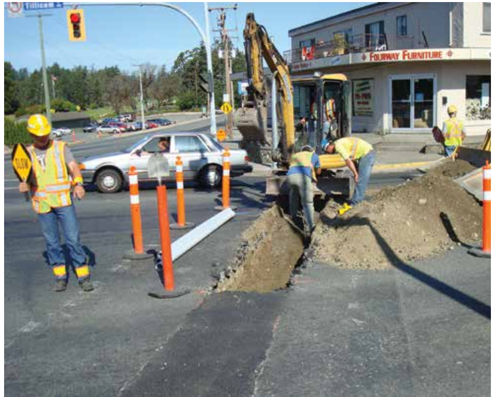
>> Installation of a conveyance pipe in Esquimalt.
