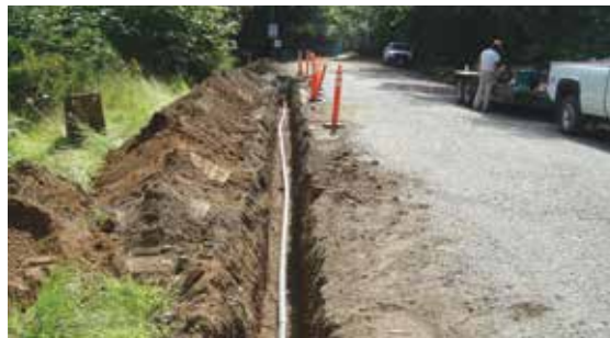
>> Pipe installation on Lambourn Drive.
