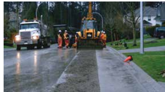
>> Trench backfilled with gravel prior to final restoration.
