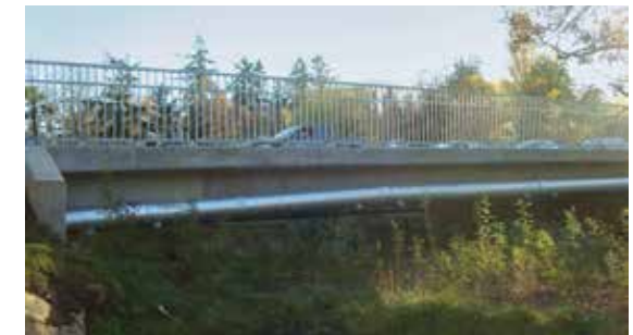
>> A sewer pipe crossing on Admirals Road Bridge.
