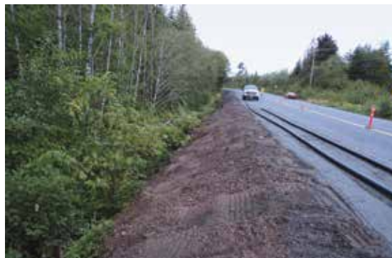
>> Installation of a conveyance pipe in Port Hardy.
