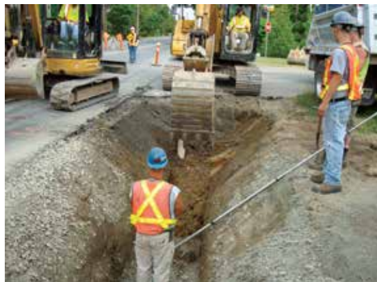
>> Installation of a conveyance pipe in Esquimalt.
