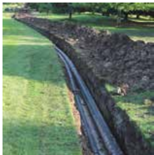
>> Typical twin-pipe common-trench installation.
