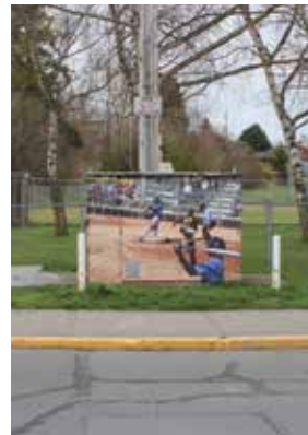
>> Lampson Street Pump Station
