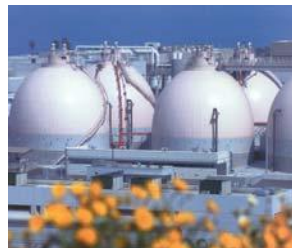
Figure 3-3 Typical Anaerobic Digesters
