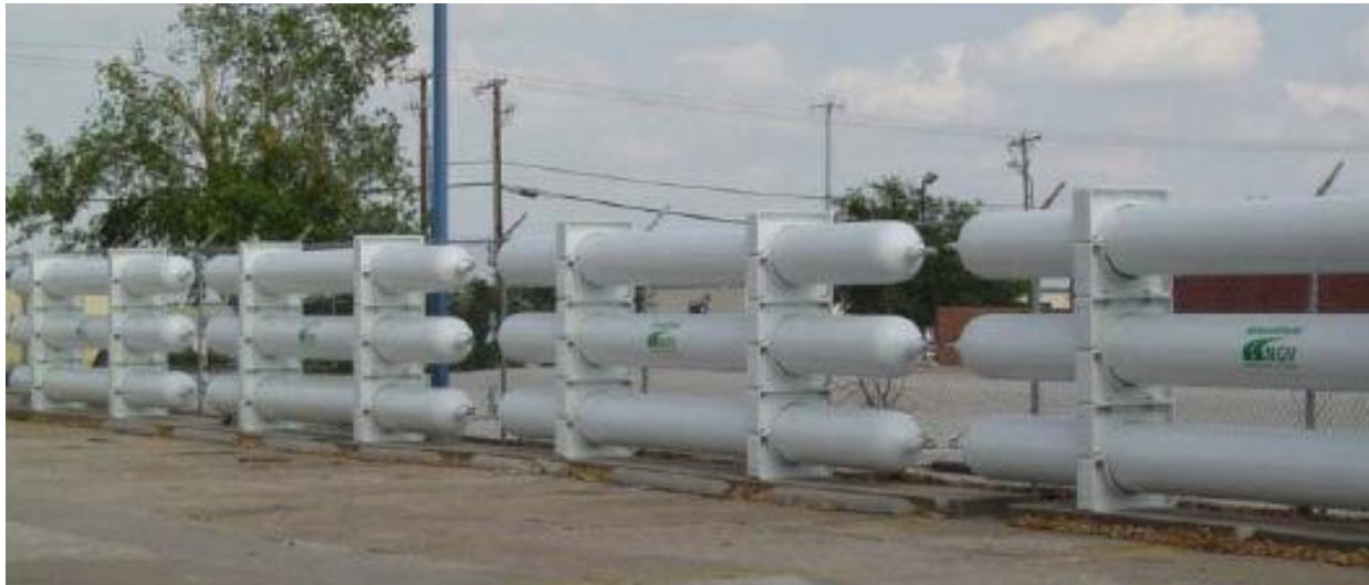
Figure 6.6 – Compressed Gas Storage Cylinders
