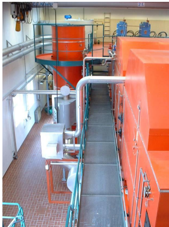
Figure 5.6 – Belt Dryer, Randers, Denmark
