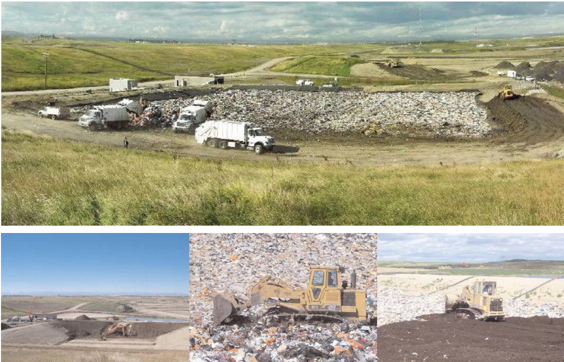
Figure 3.13 – Biocell in Operation (Stantec, 2006)
