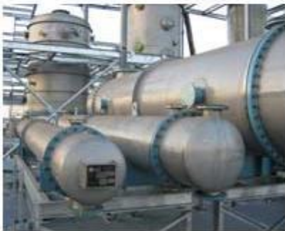
Figure 10.2 Diagram and Photos of Shell and Tube Heat Exchangers
