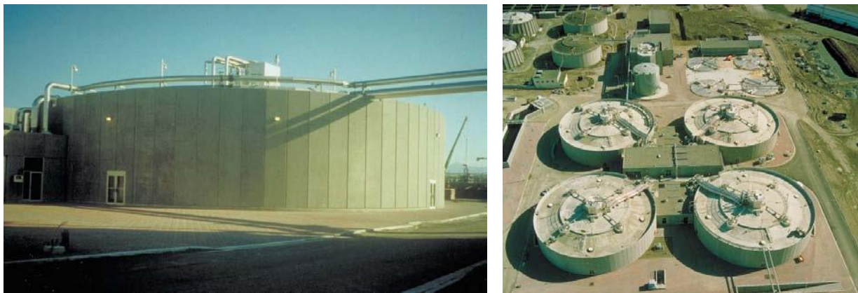
Figure 5.3 – Thermophilic Anaerobic Digesters: Metro Vancouver’s Annacis Island WWTP
