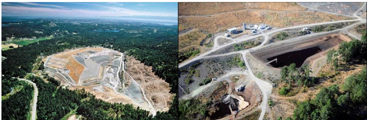
Figure 3.23 – Overview of Landfill Area (left) and Gas Utilization Facility and Leachate Collection Ponds (right)
