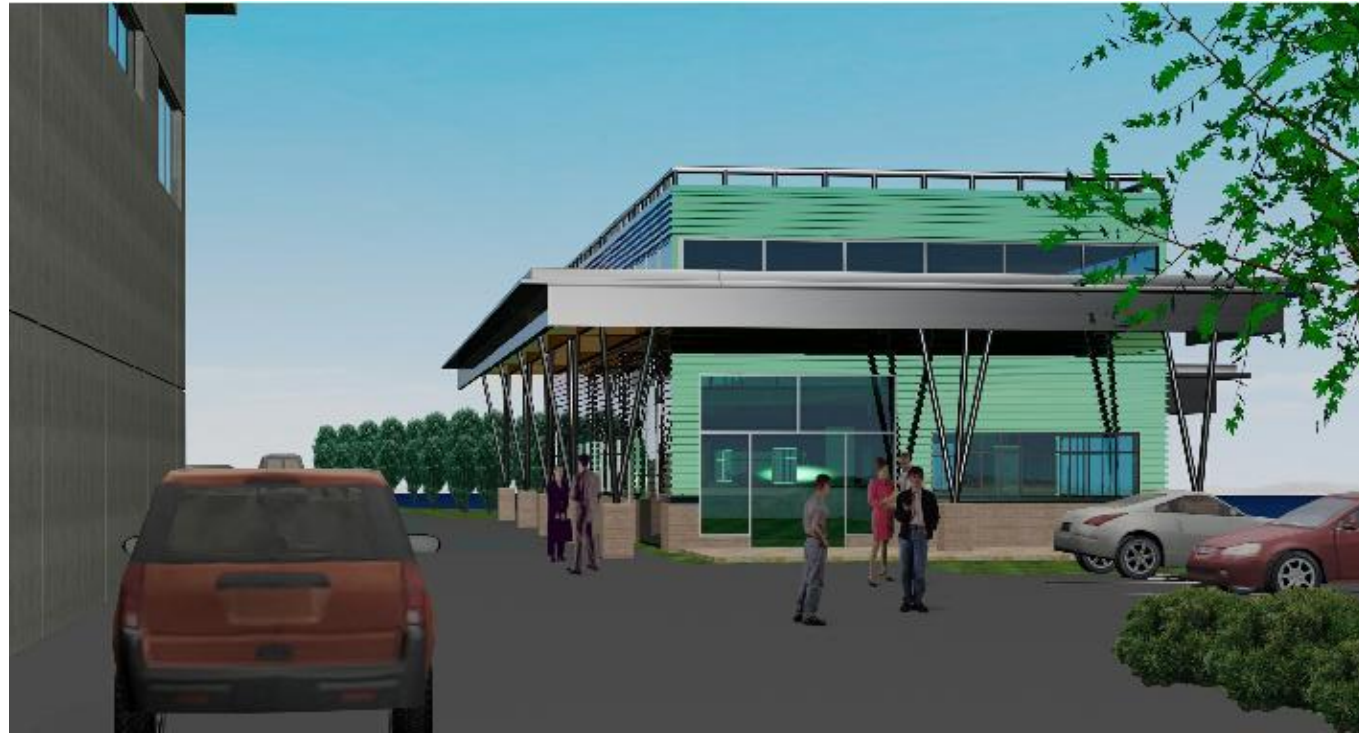
OPERATONS BUILDING (LOOKING NORTHWEST)
