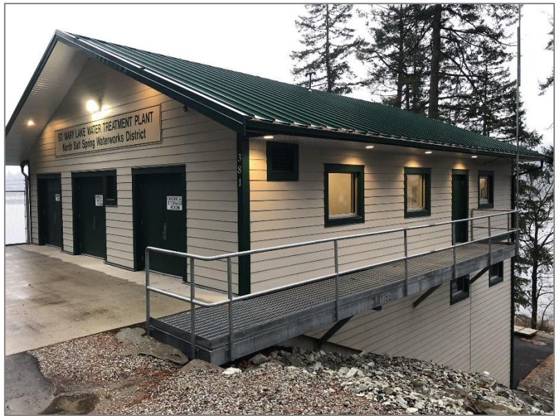
Figure 2-3 NSSWD St. Mary's Treatment Plant
