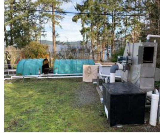
RBC Units, Screen, and splitter box
