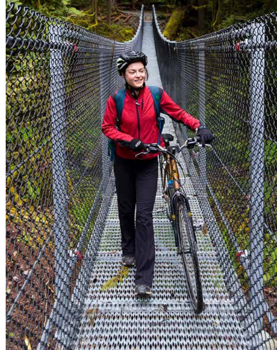
3 km from the south trail head is Goldstream River suspension bridge. Click to watch a time-lapse video of the bridge construction.
