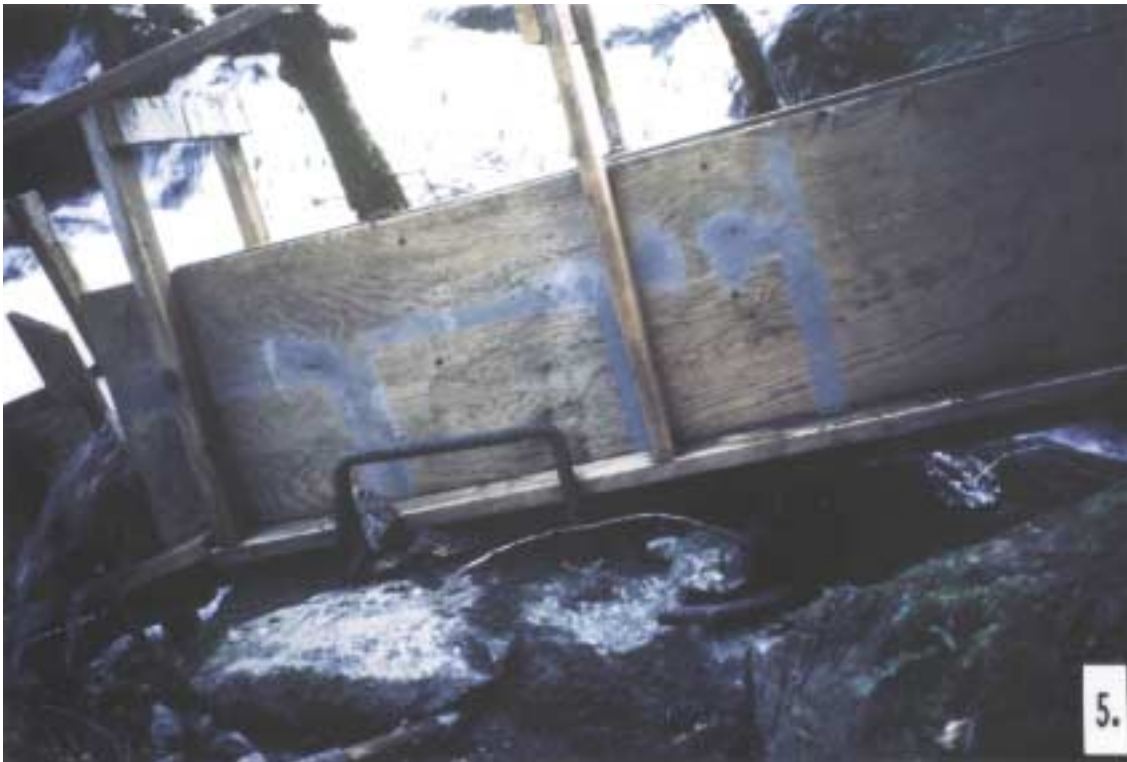
Remnants of naval flume
