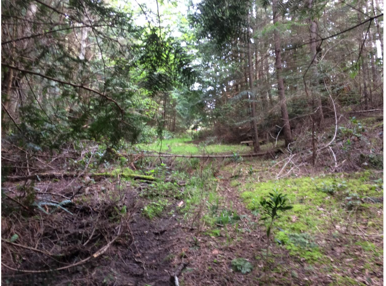
Photograph 9. Along the channel upstream from Harbour Hill Drive
