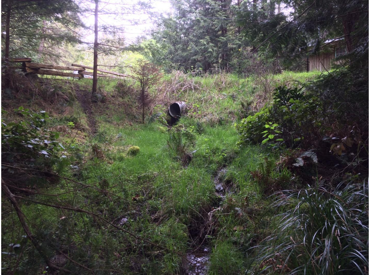
Photograph 8. Looking north at the culvert under Gardam Lane. The sedges on the right of the picture indicate that this is a water catchment area. The area beneath the culvert is suitable for a small pool.
