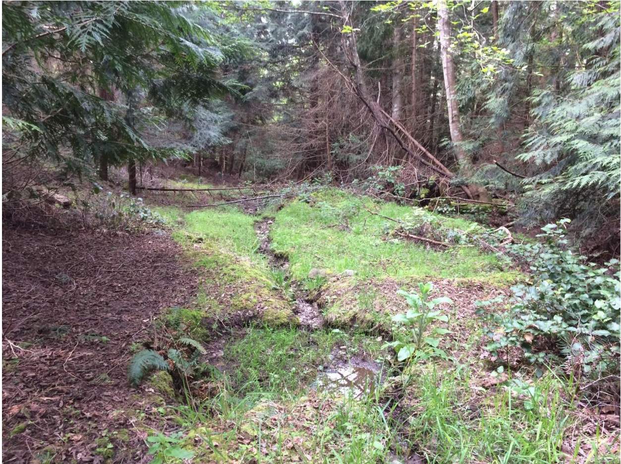
Photograph 7. Looking downstream from the culvert on Gardom Lane
