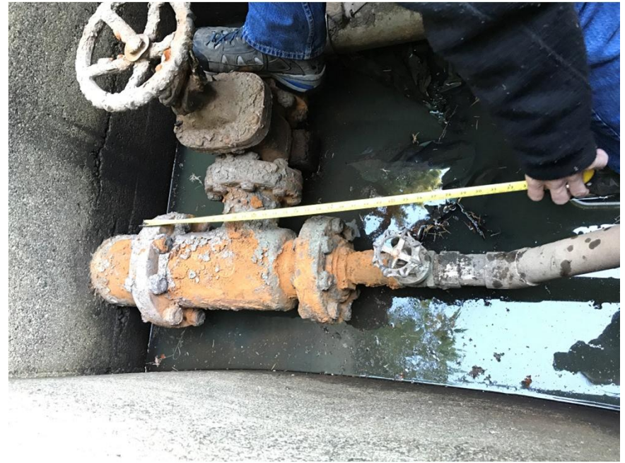
Photograph #2 – Top View: Low Level Outlet Chamber Infrastructure Deposit build-up partially removed
