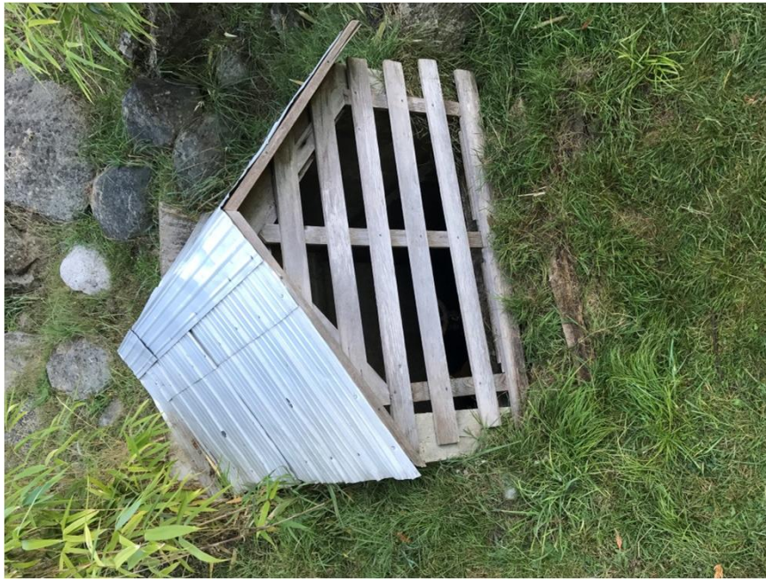
Photograph #1: Low Level Outlet Chamber and Housing Located on downstream face of Gardom Pond Dam
