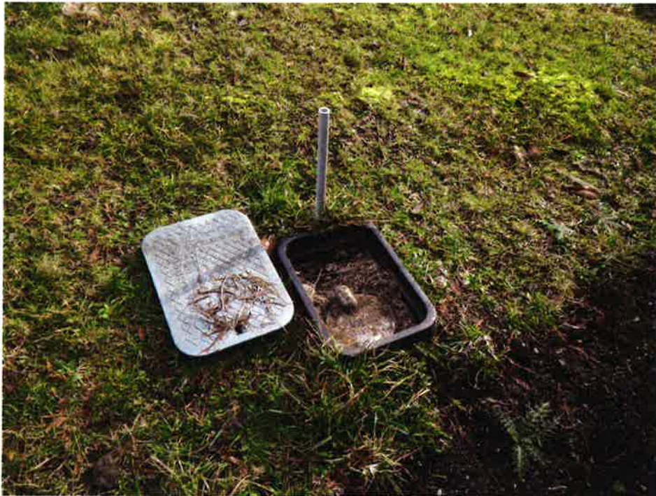
Photo 9: Valve cover for nearby well (Feb. 13, 2013).
