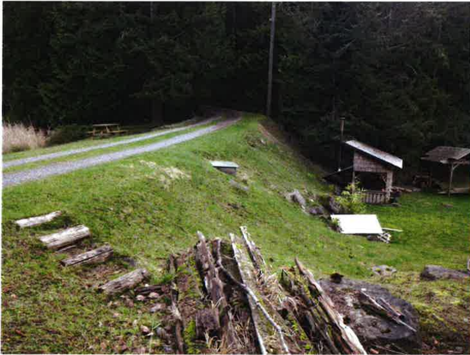
Photo 1: Gardom Pond Dam from right abutment (Feb. 13, 2013)
