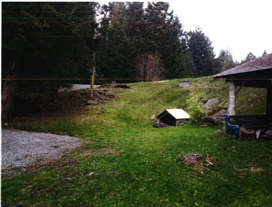
Photo 4: Area below downstream slope (Feb. 13, 2013).
