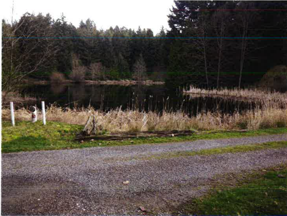
Photo 7: Gardom Pond from right abutment area (Feb 13, 2013)
