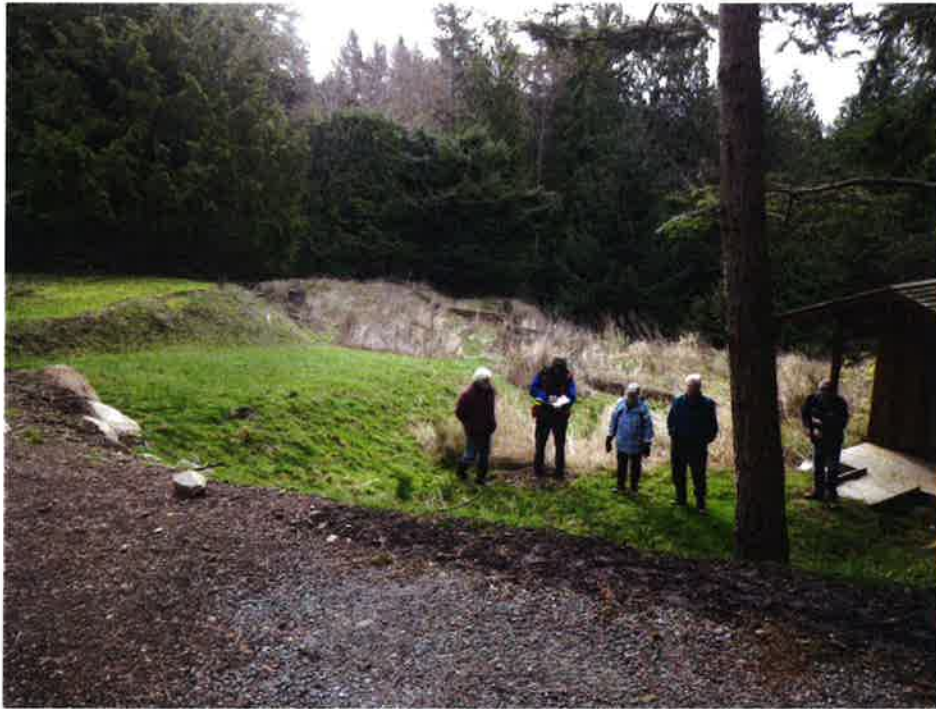
Photo 5: Area downstream of dam – note terracing (Feb. 13, 2013).
