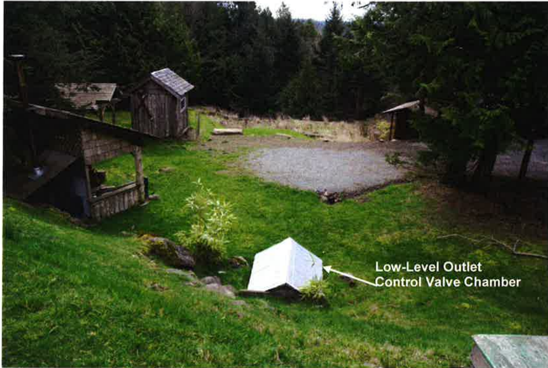
Photograph #3 – Looking Downstream from Dam at Centreline of Crest
