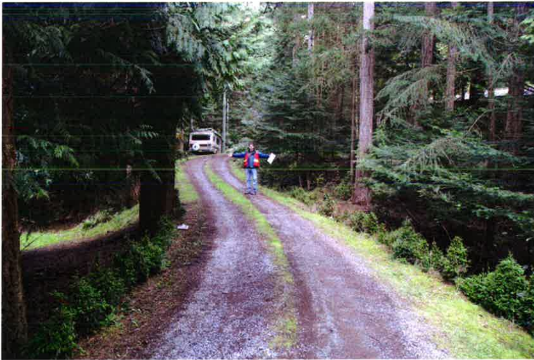
Photograph #10 – Possible Location of New Spillway beneath Gardom Lane (from left to right)
