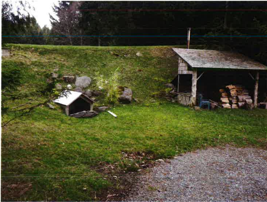
Photo 3: Area below downstream slope. Note outlet chamber and boulder stack.
