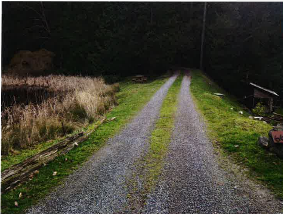
Photo 2: Looking east along dam crest from right abutment (Feb. 13, 2013)
