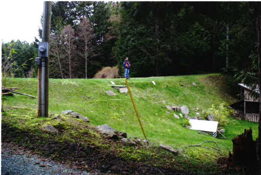
Photograph #4 – Downstream Face of Dam
