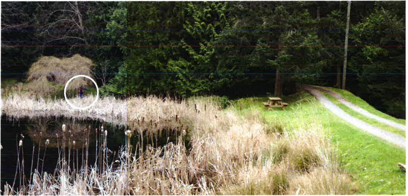
Photograph #9 – Proposed Site of New Spillway (engineer standing at location)
