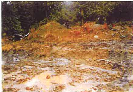
Right Abutment - December 1, 1977
