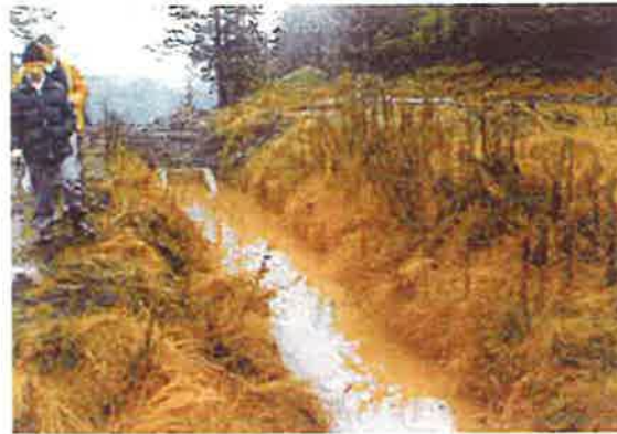
Intake Channel - December 1, 1977
