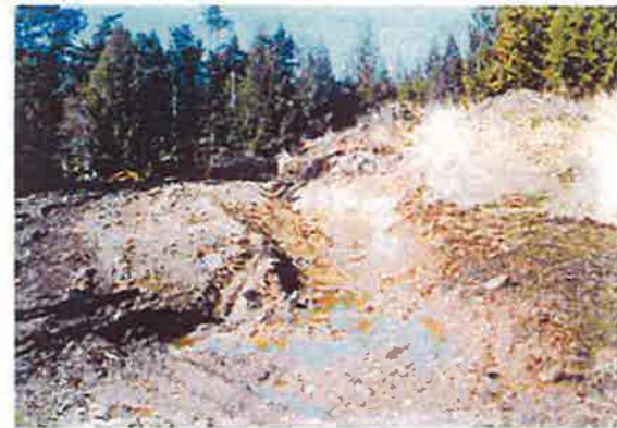
Spillway Cut Viewed From Upstream End - March 20, 1977
