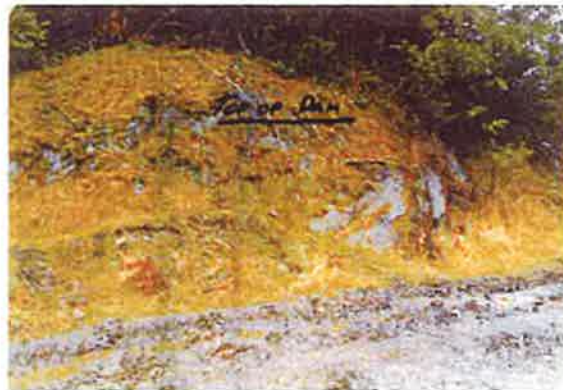
Left Abutment - December 1, 1977
