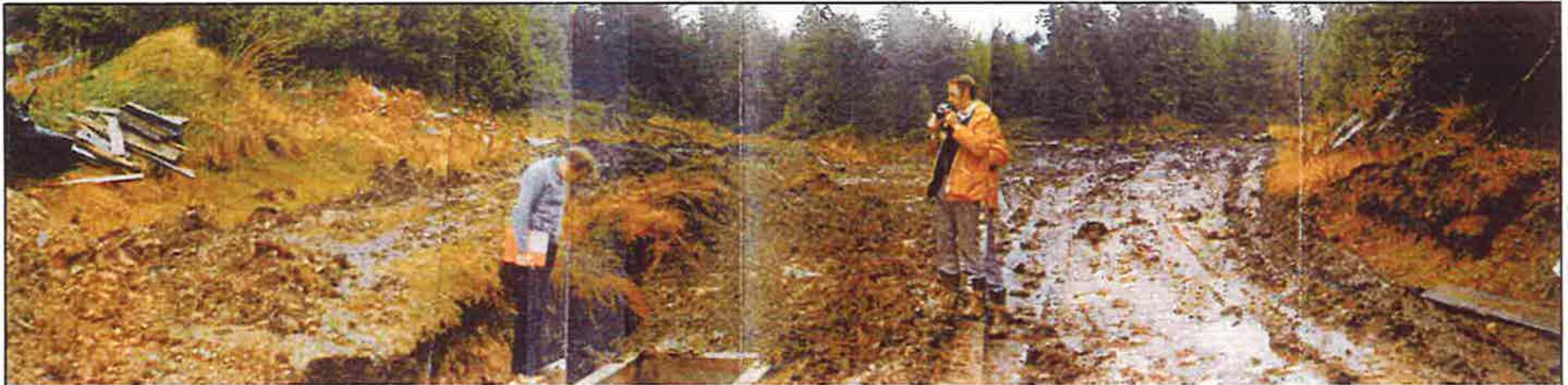
Panorama Centered Over Sluice Trench - December 1, 1977
