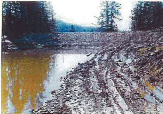
Downstream Face of Dam - March 20, 1979
