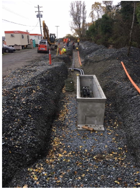
Figure 5 – Installation of BC Hydro ductbank
