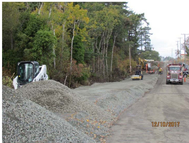
Figure 3- Widening of Victoria View road
