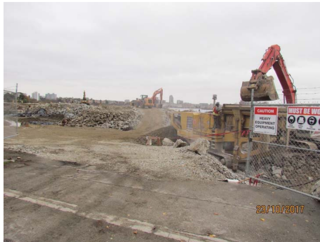
Figure 2 — Crushing of blast rock
