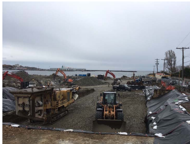
Figure 6 – Slope stabilization and protection
