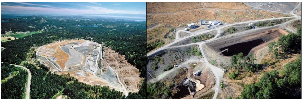
Figure 3.23 – Overview of Landfill Area (left) and Gas Utilization Facility and Leachate Collection Ponds (right)
