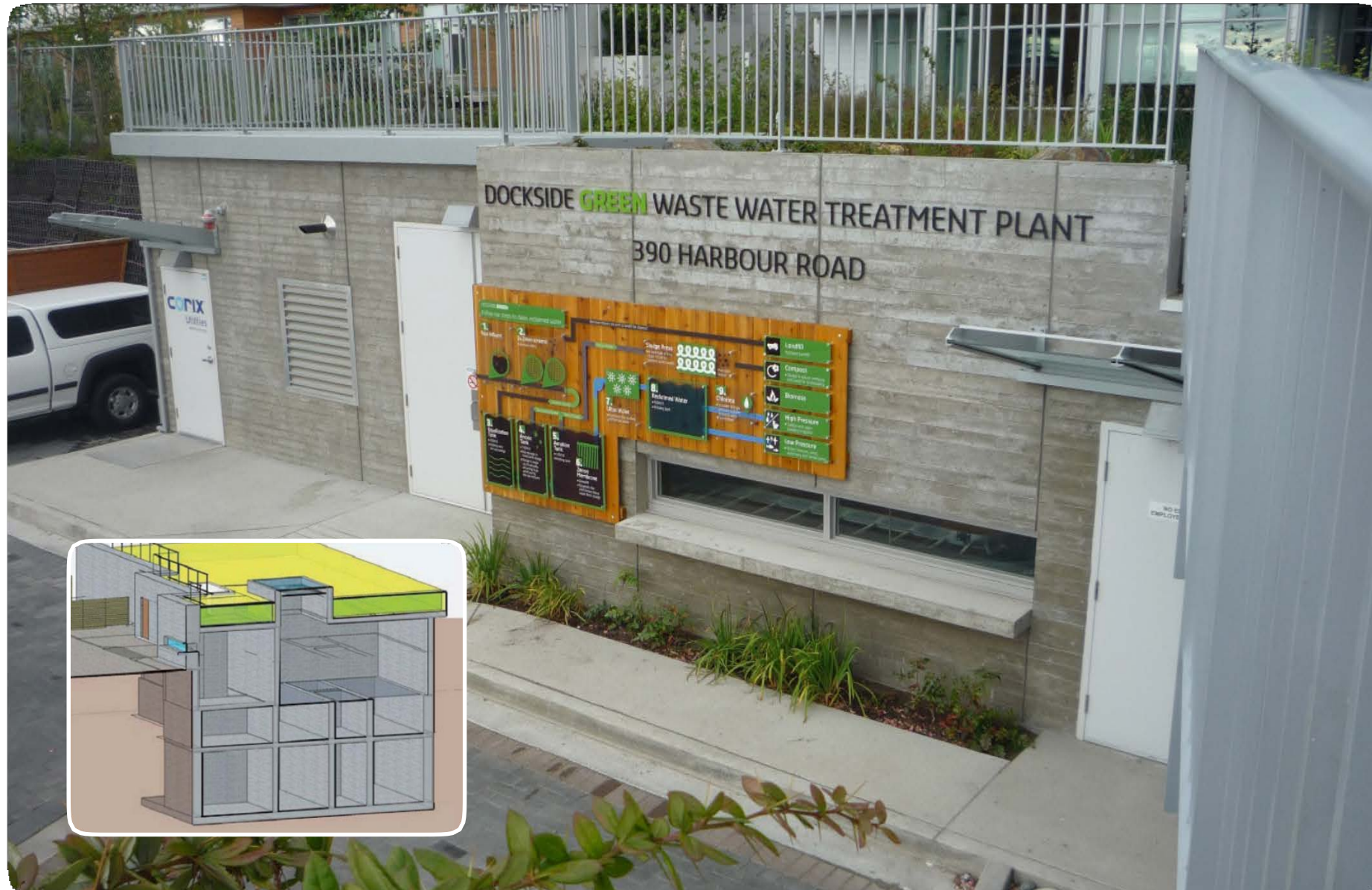
Waste water treatment plant
