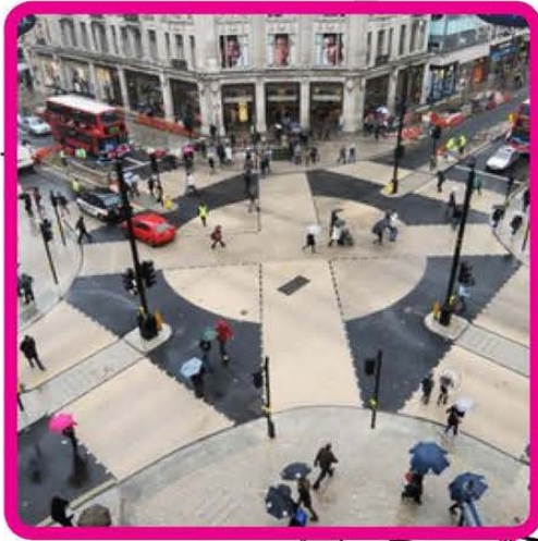
Put in a scramble intersection such as the Oxford Circus where a busy vehicular street takes time for pedestrian crossings during peak walking hours.
