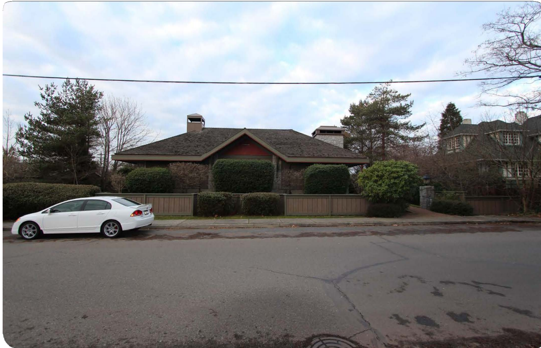
Currie Road Wastewater Pump Station
